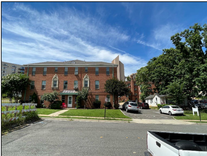
Figure 7. View of Existing Wakefield Manor from Fairfax Drive
