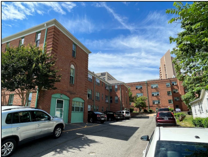
Figure 6. View of Existing Wakefield Manor from Fairfax Drive
