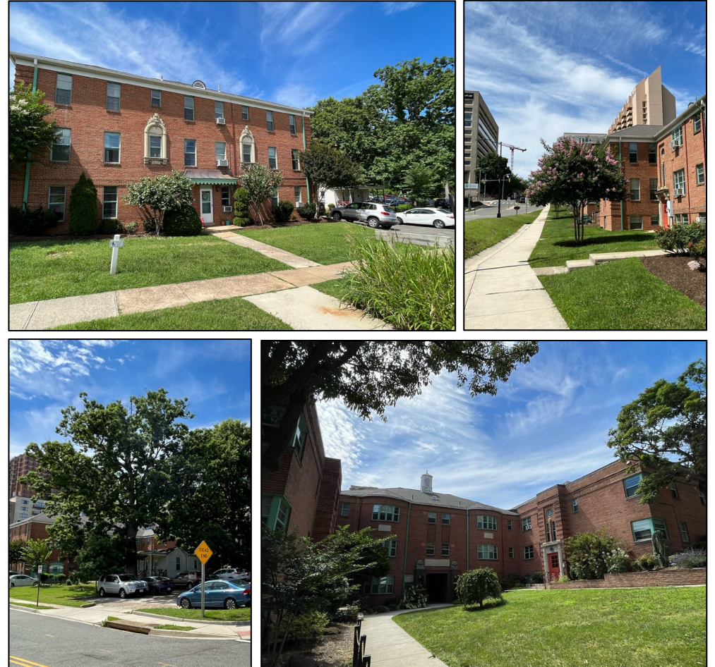
Existing site photos
