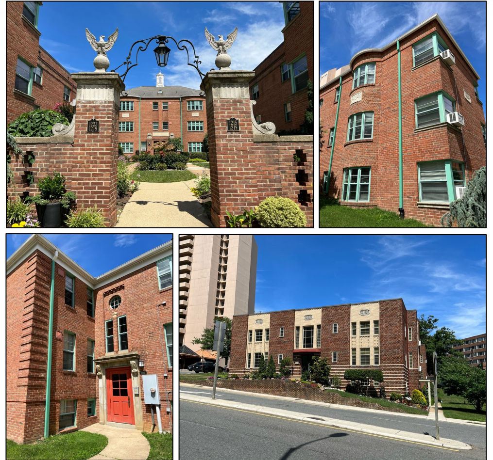
Existing site photos
