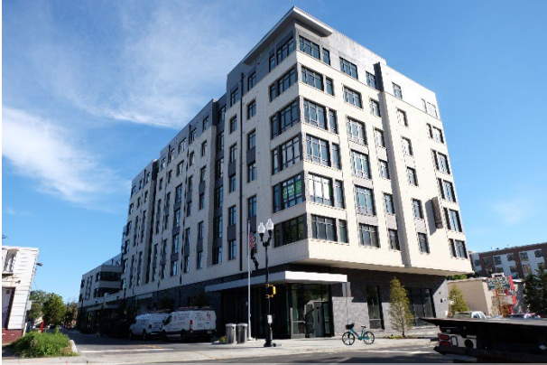
Terwilliger Place – view looking northeast
