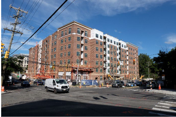
Mill Creek Residential – view looking northwest
