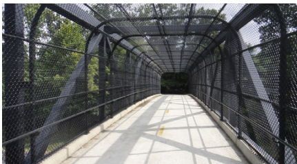
Bethesda Trolley Trail Bridge, MD
