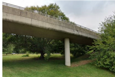
Existing MVT bridge crossing
