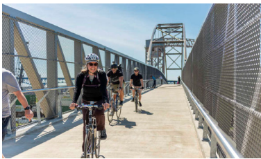
Wendy Park Bridge - Cleveland, OH
