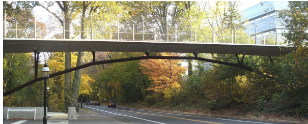
Streicker Bridge - Princeton, NJ
