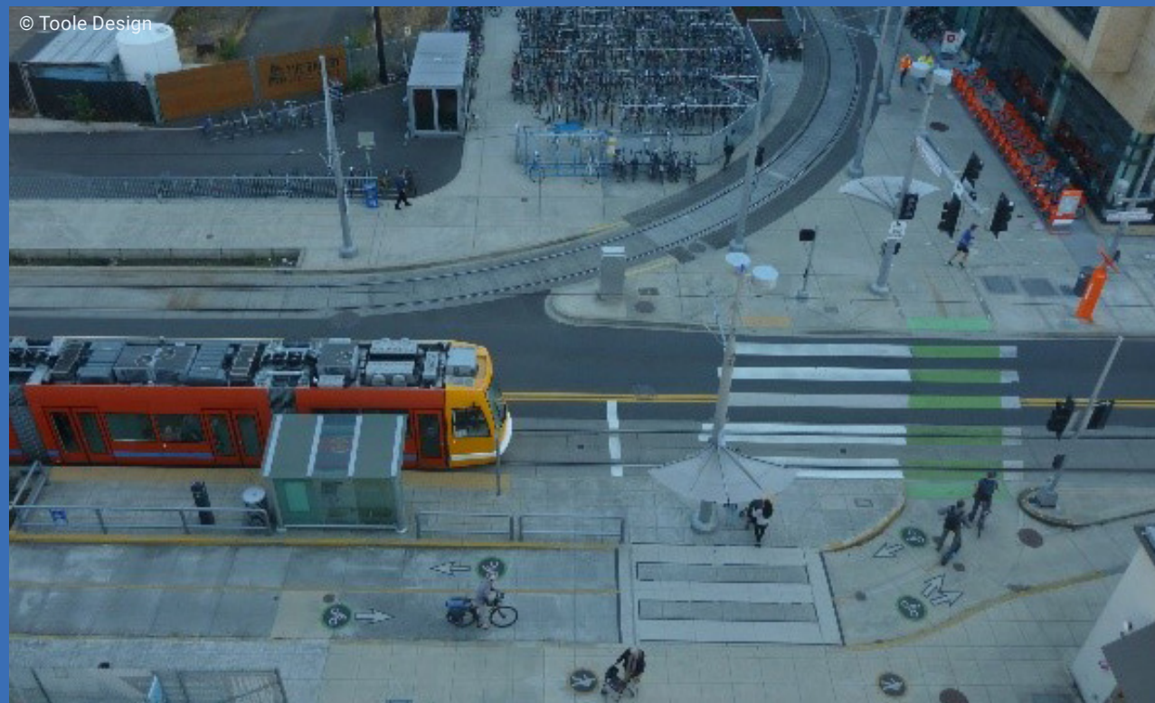
Figure 3 South Waterfront Lower Tram Terminal Gateway Mobility Hub, Portland, OR
