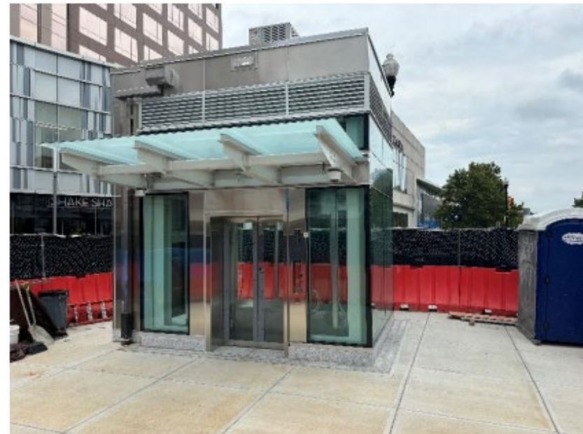
New elevator located at 12th Street S and Hayes Street
