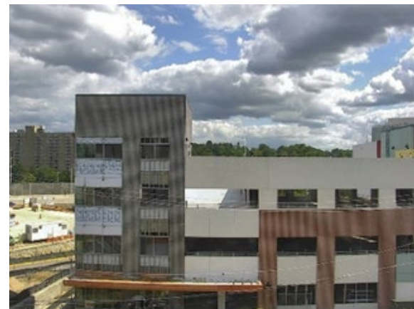
New O&M facility (top) and new garage (bottom)
