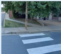
**Safety Issue:** The crosswalk leading to St. Agnes School was not marked or ADA accessible. Previously, there was a crosswalk on N Randolph St that led directly to a utility pole and did not have a curb ramp.
