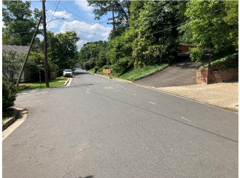
Figure 2: Looking South at the intersection of 17th Street S.
