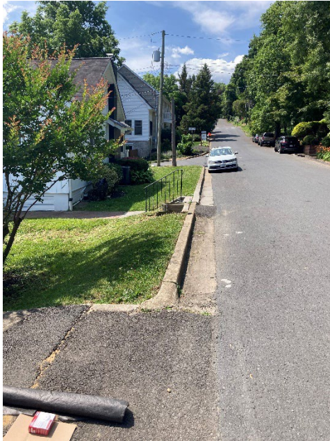
Figure 1: Looking South at the intersection of 19th Street S.
