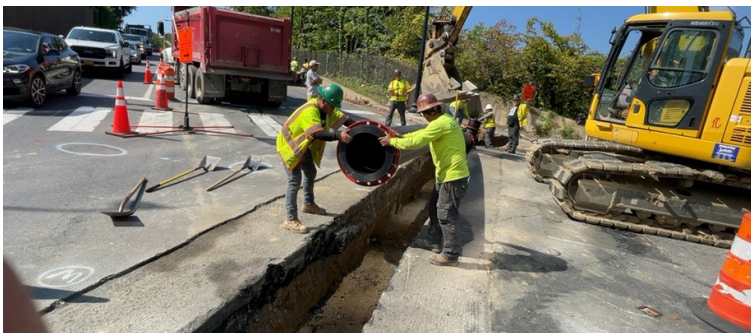
Temporary bypass placed on Langston Boulevard and I-66.
