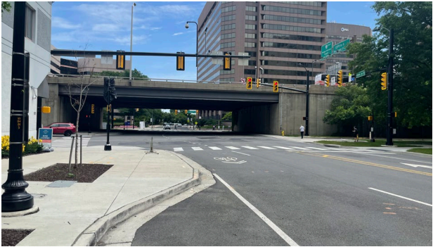
12 th Street South Improvement (S. Eads St. – S. Clark St.) ($4.2M)
