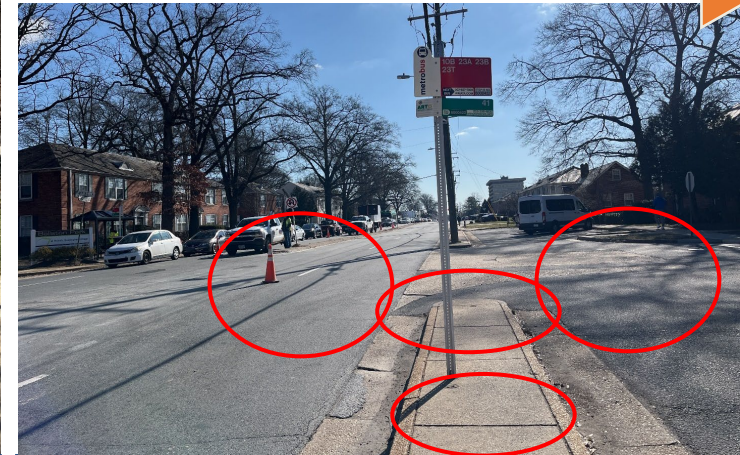
Compliance = widen sidewalk/pad, curb ramps, crossings, regrading
