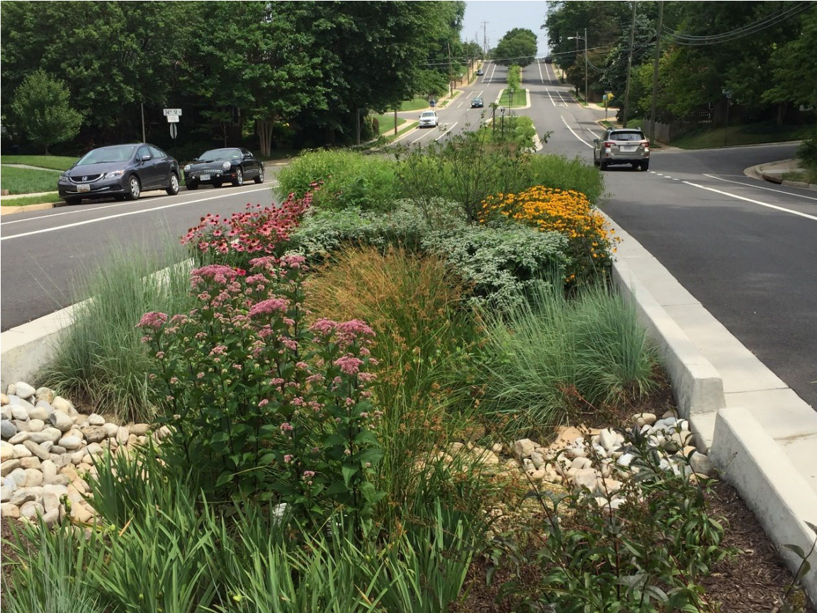
Newly planted bioretention plants at the Williamsburg Green Street project (Planted May 2018)
