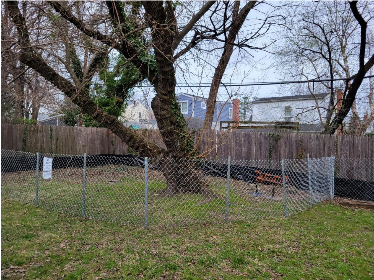
4 Ft Chain Link Fence – Example 2 – Open grown tree with partial CRZ protection
