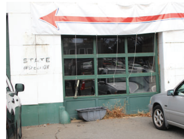
Figure 015 Detail of garage bay doors. EHT Tracerics, August 2019.
