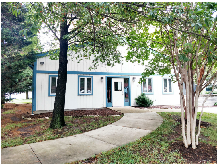
7) EXISTING STRUCTURE TO THE EAST OF THE PROJECT SITE.
