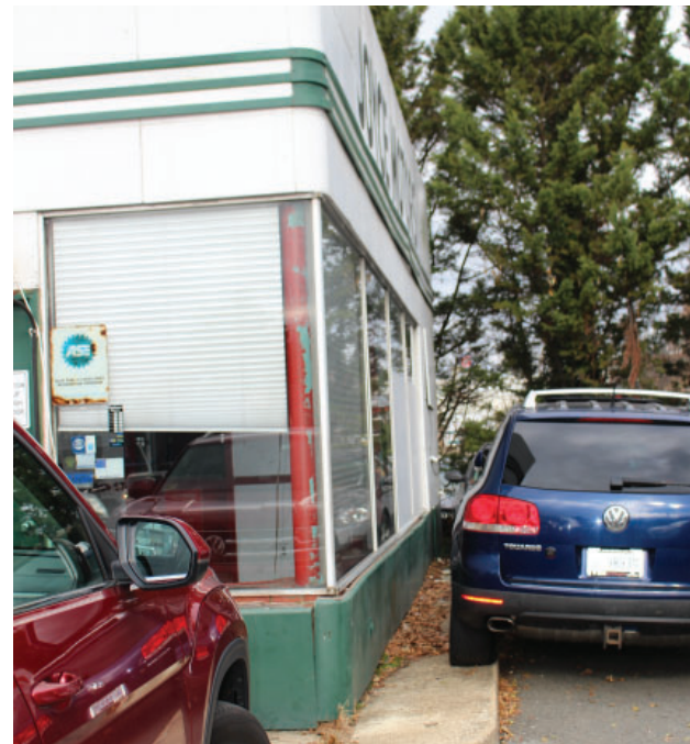
Figure 004 Detail of structural glass walls. EHT Tracerics, December 2018.
