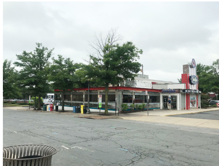
5) SILVER DINER BUILDING TO THE NORTH OF PROJECT SITE. VIEW FROM INTERSECTION OF WASHINGTON BLVD AND N IRVING STREET.
