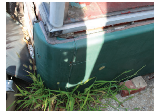
Figure 017 Detail of green porcelain enamel panels with rounded corner. EHT Tracerics, August 2019.
