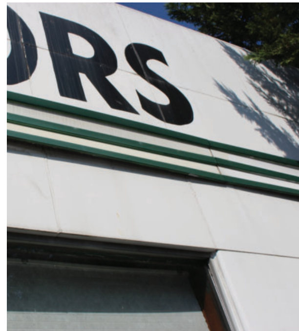
Figure 003 Detail of porcelain enamel panels. EHT Tracerics, December 2018.
