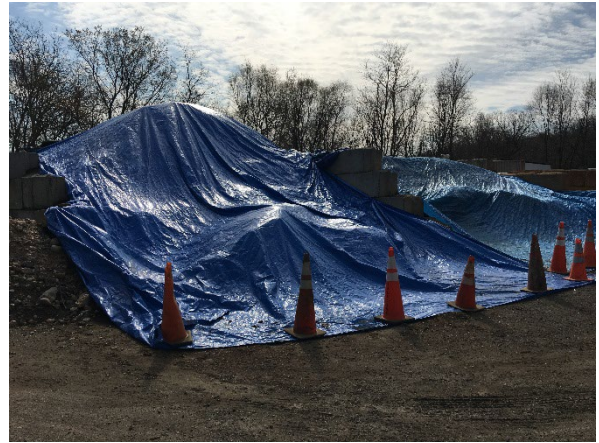
Photo 2: Covered bulk material storage area
