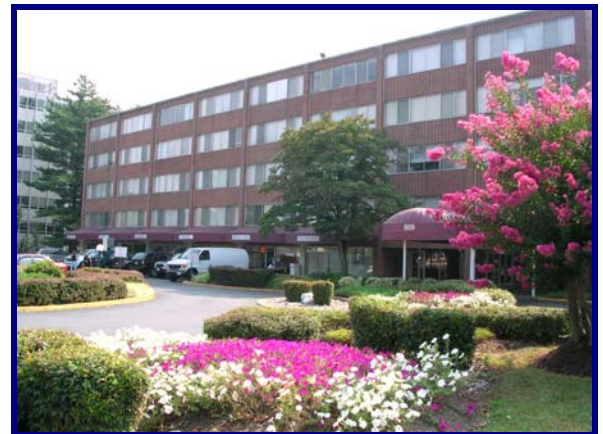
Broad Falls Apartments
