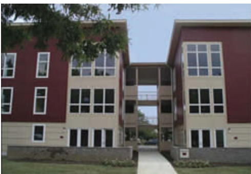
Davis Place, a new construction Affordable Dwelling Unit development in the Nauck Neighborhood Strategy Area.
