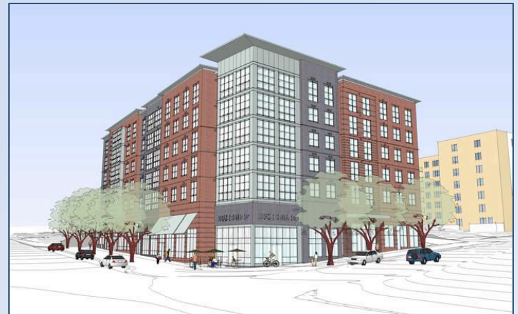
The Shell (under construction)
