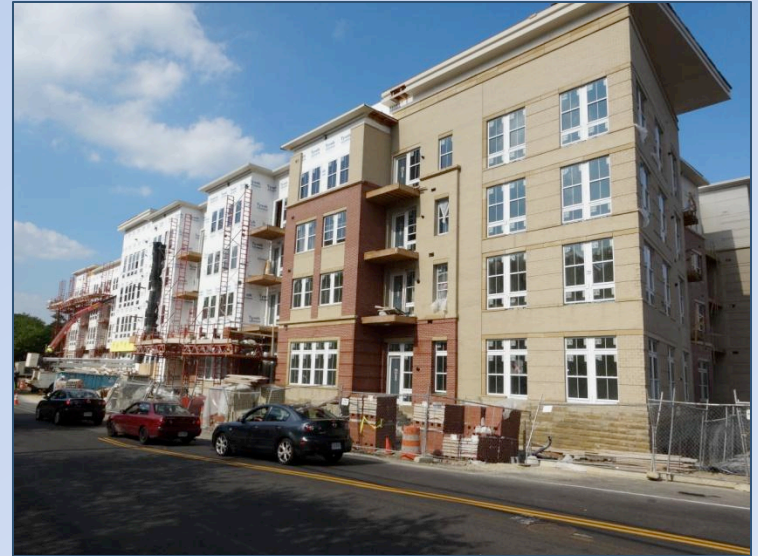
Arlington Mill (under construction)
