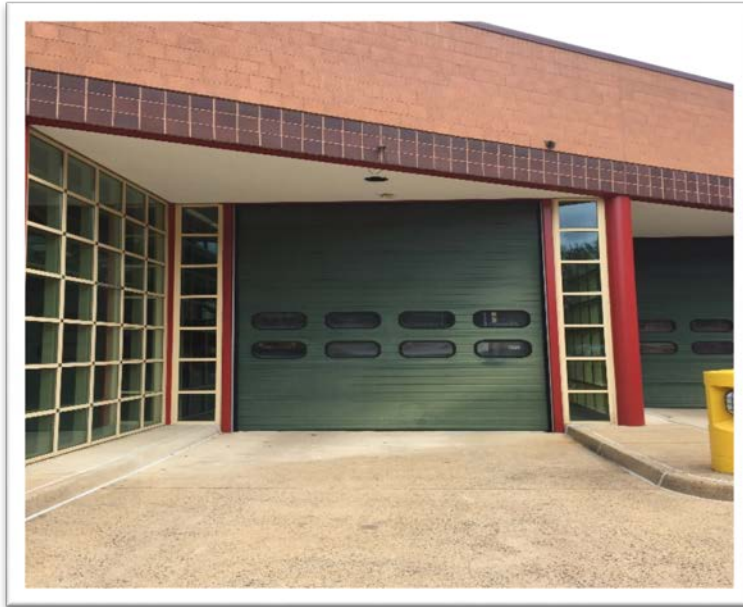
Original Overhead Doors
