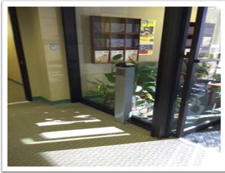
Automatic Door Opening System
