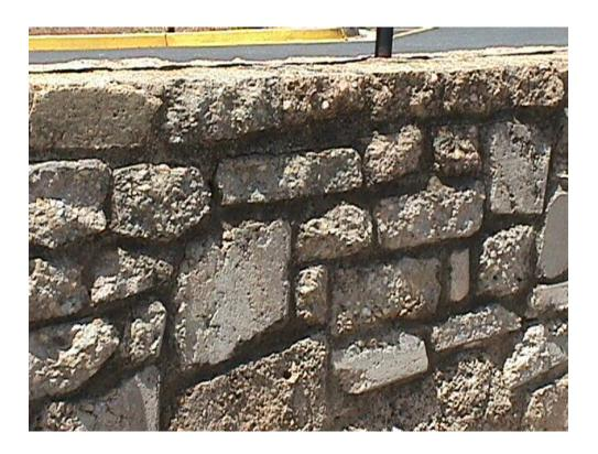
Below is a photo of a County Standard, DPW built stone faced rubble retaining wall installed next to a park along Lorcom Lane. Maintenance is by the County.
