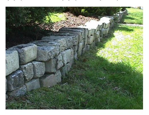
Below is a photo of a County Standard, DPW built mortar rubble retaining wall installed next to the parking lot at Swanson Middle School. Maintenance is by the County.
