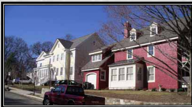
Cherry Hill Five houses at 18 th Road and N. Randolph Street
