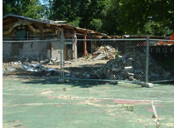
The Walter Reed Rec Center being demolished (2004).
