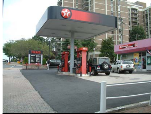
The Texaco Station was installed during the same era as Bob & Edith's Diner.
