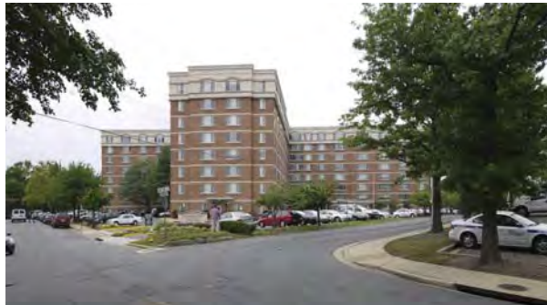
Existing Conditions, Dominion Plaza Apartments
