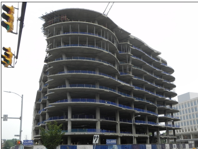
Founder's Square Under Construction - January 2011
