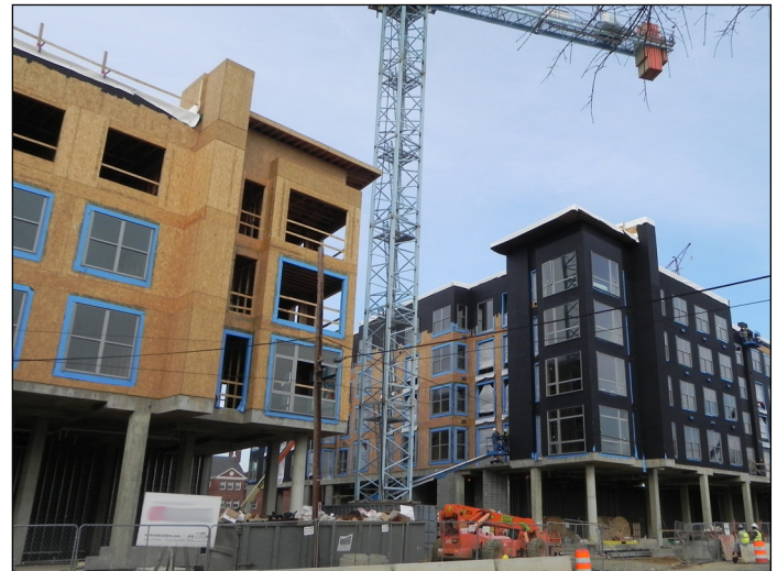
Mosaic at Clarendon Project Under Construction
