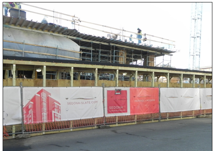
The Slate and Sedona Project Under Construction
