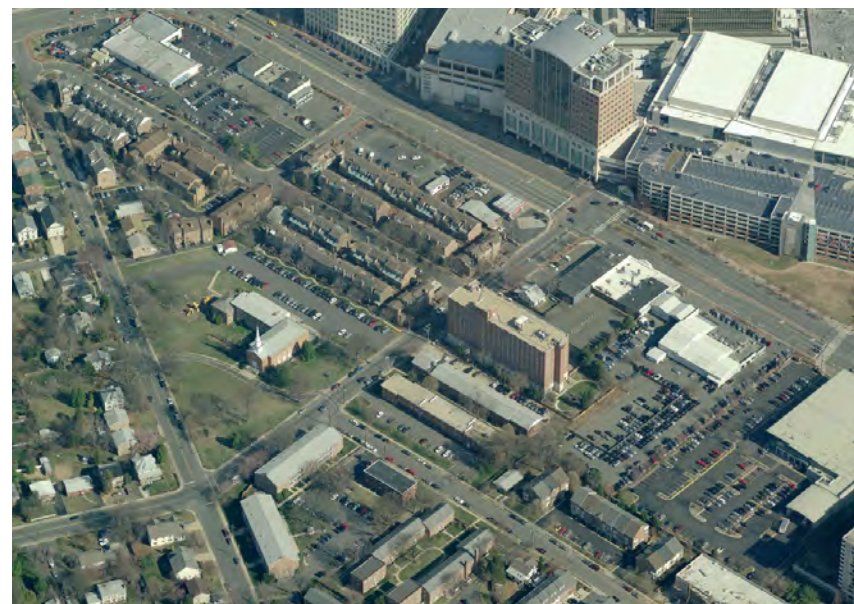
Aerial photo of West Ballston area (2009)
