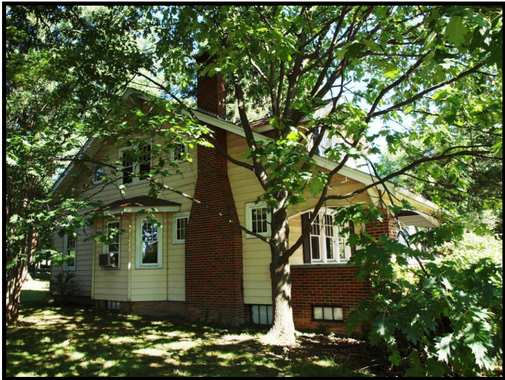
Photo 11: South side elevation of the Fraber House, facing northwest.
