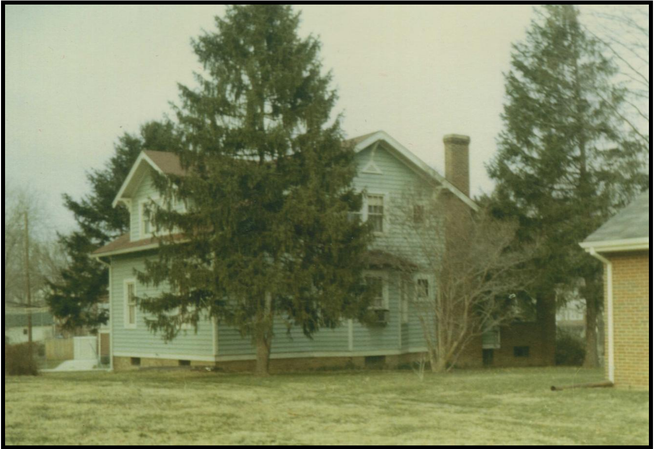
Photo 7: The south (rear) and west elevations of 1612 North Quincy Street, sometime in the 1950s when the original ivory siding was painted blue. The original wood brackets are visible along the eaves and the house remains virtually unchanged. The brick rambler, which replaced the 19 th -century farm house at 1608 North Quincy Street, is visible at the far right.
