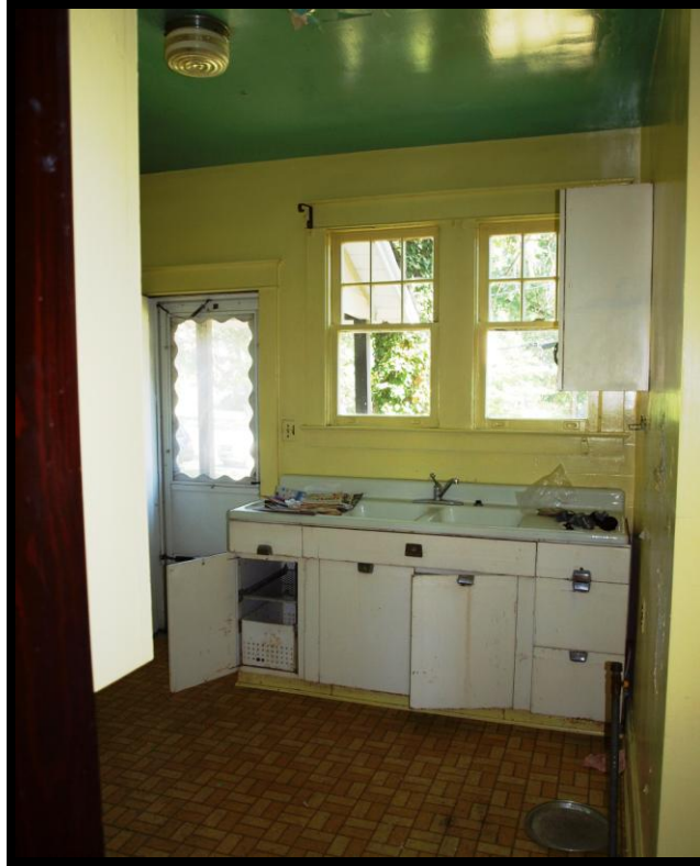
Photo 16: View of kitchen, with original cast iron sink and replacement metal cabinets, facing north.
