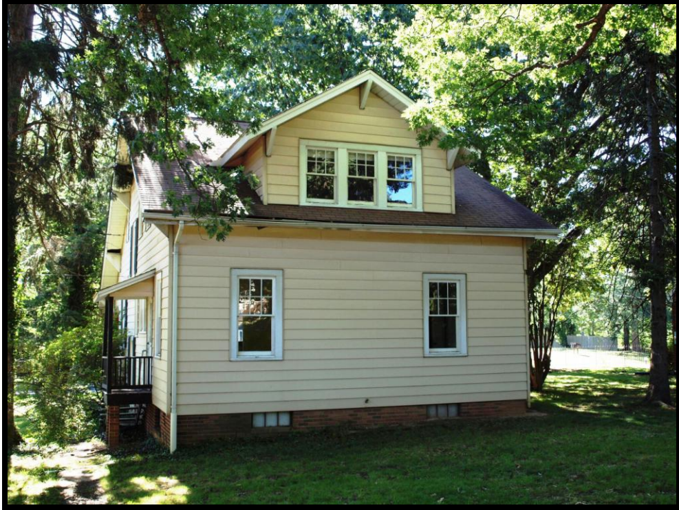
Photo 10: West (rear) elevation of the Fraber House, facing east.
