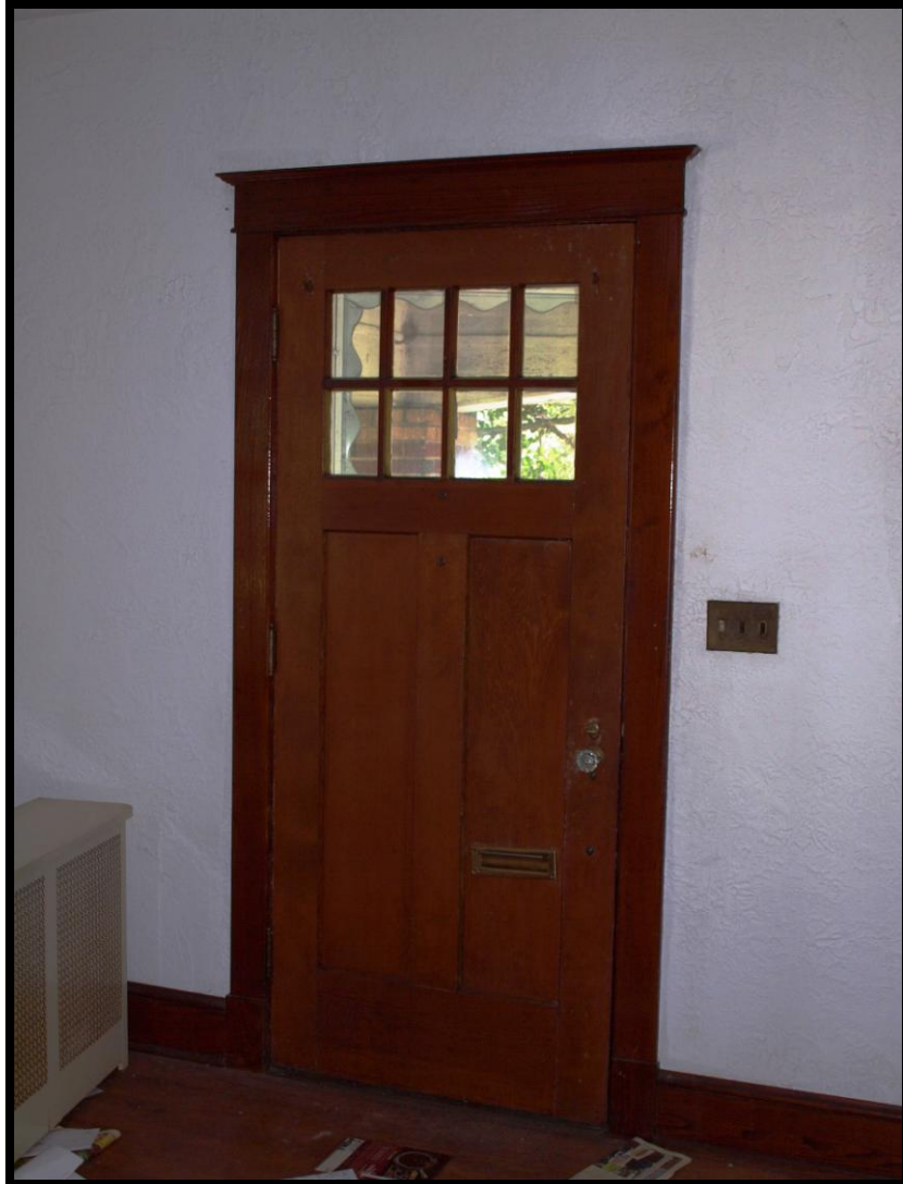
Photo 12: Interior view of the original front door.
