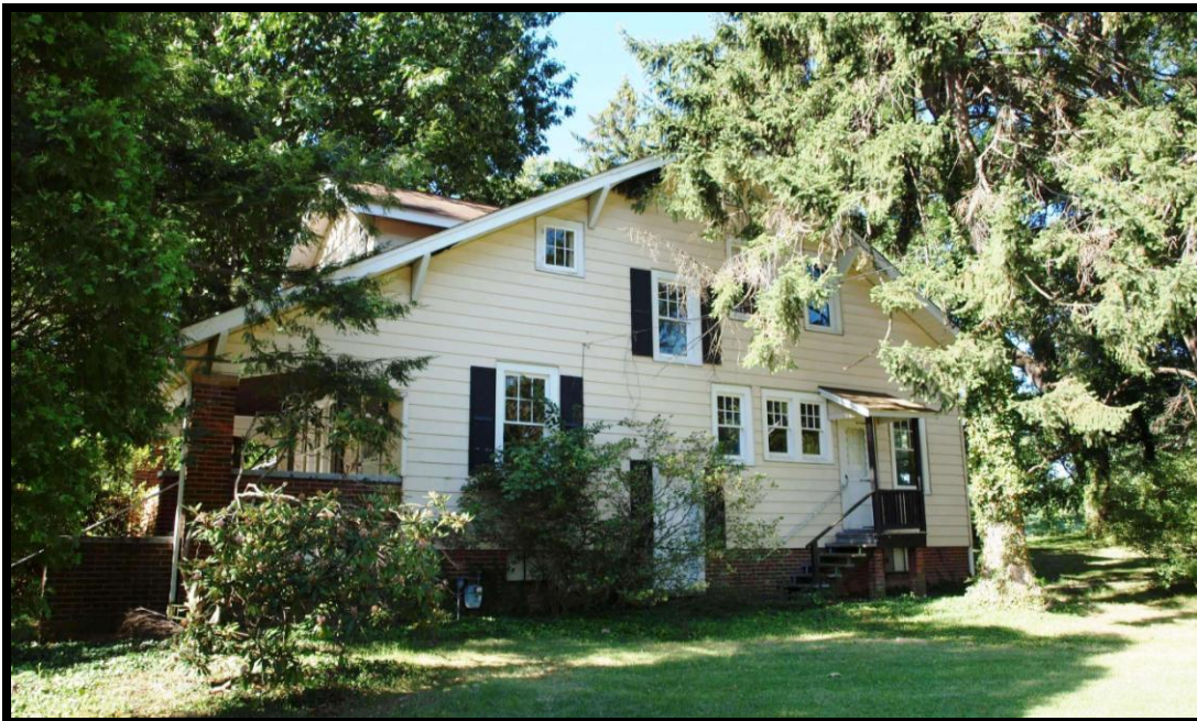
Photo 9: North side elevation of the Fraber House, facing southwest.
