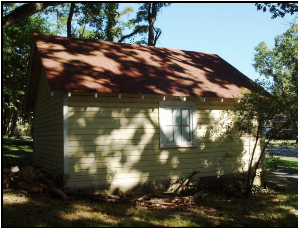
Photo 24: East and south elevations of the original garage.
