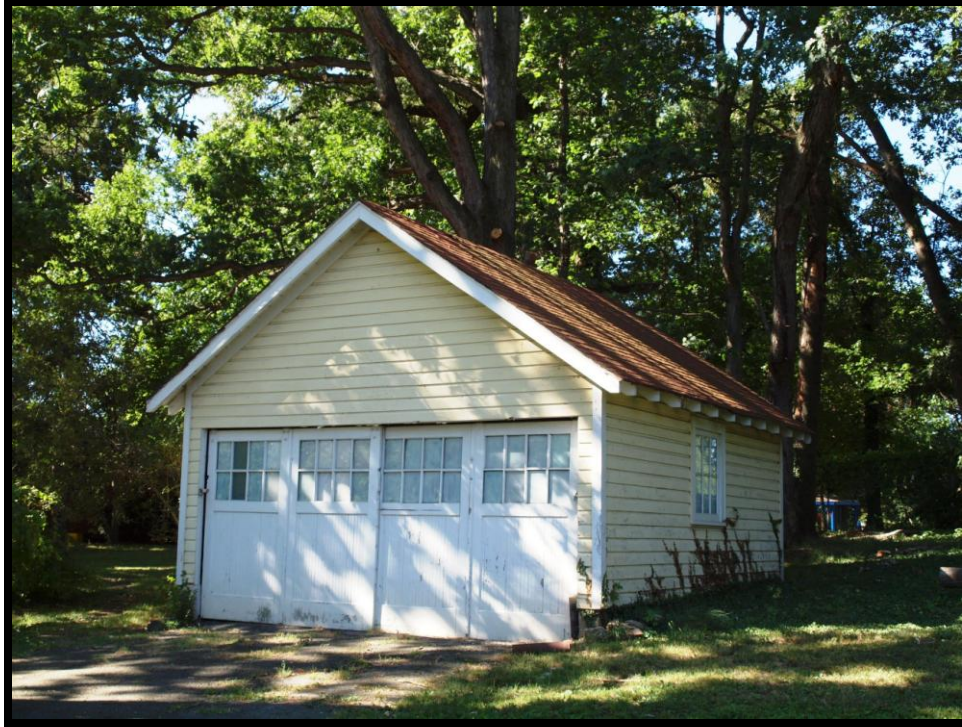
Photo 23: North and west elevations of the original detached garage at the Fraber House. Note the original drop wood siding, doors, and windows.
