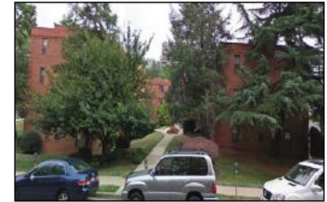
Queens Court Apartments
