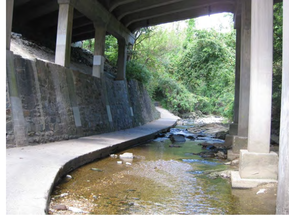
Under Four Mile Run bridge
