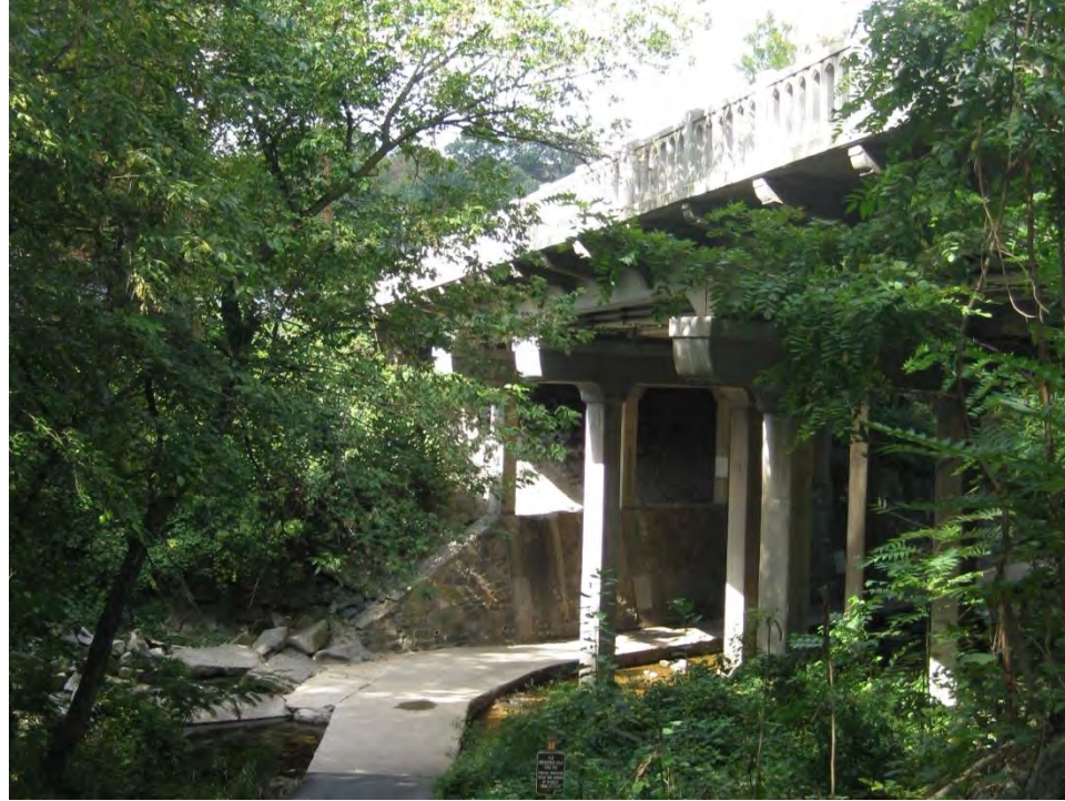
Four Mile Run bridge (looking northwest from Four Mile Run Trail)
