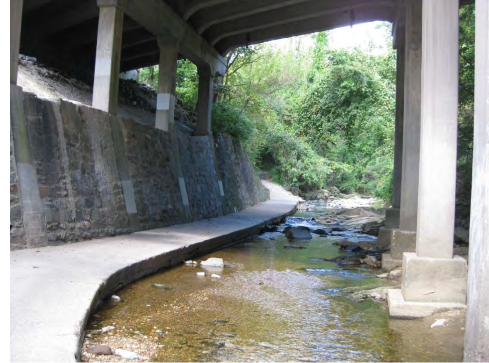
Under Four Mile Run bridge
