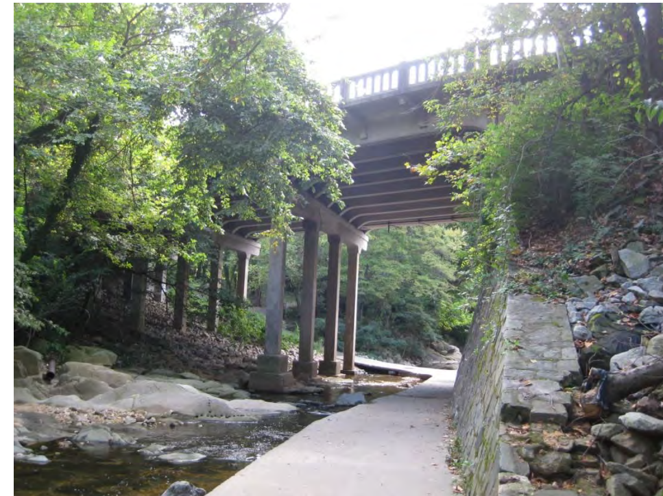
Four Mile Run bridge (looking southwest from Four Mile Run Trail)
