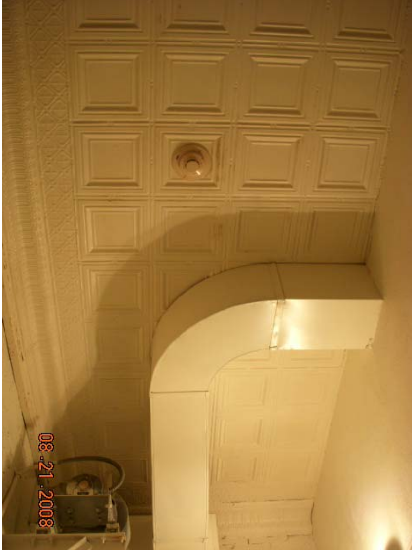
Figure 6: Detail of original pressed tin ceiling visible in second floor hall closet. Image courtesy of the Arlington County Historic Preservation Program, August 2008.
