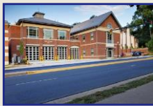
Fire Station #3 – Old Dominion Dr
