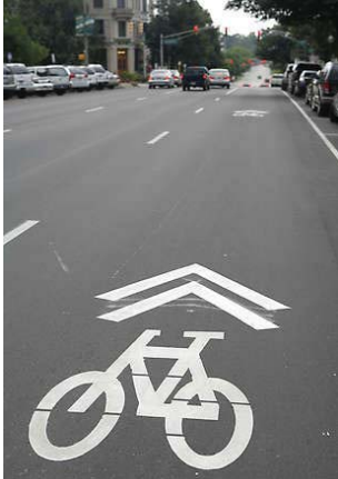
Sharrow pavement marking
