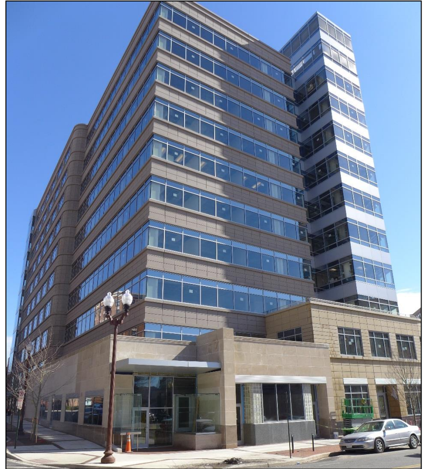
Penzance project in Clarendon, with two historic facades preserved at lower left
