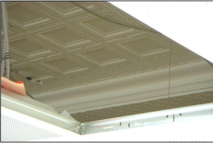
Original ceiling tiles from 1910 section of Wilson School
