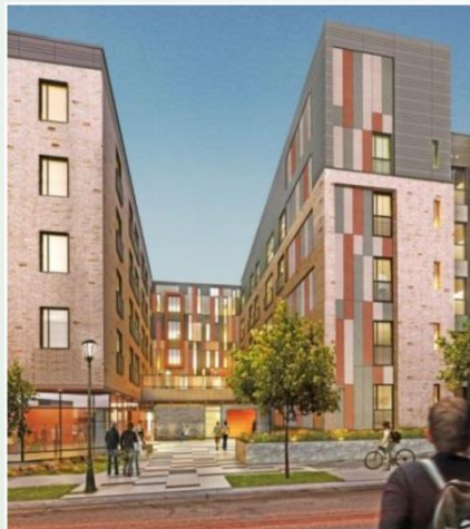
Courtyard fronting Thomas Street
