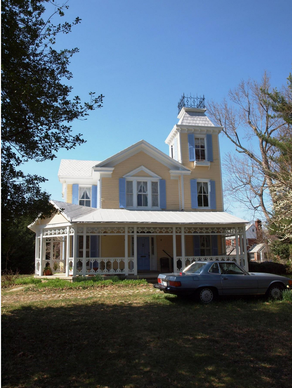
Figure 1: View of the east elevation of Broadview looking west from the neighboring lot. Historically, this elevation served as the building's front facade.
