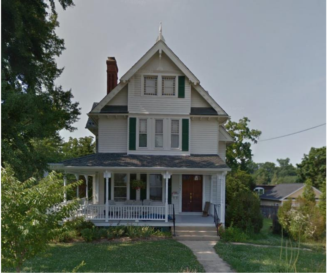
Figure 6: View of the Queen Anne-styled General Samuel S. Burdett House at 5627 3rd Street South. Source: Google, 2012.
