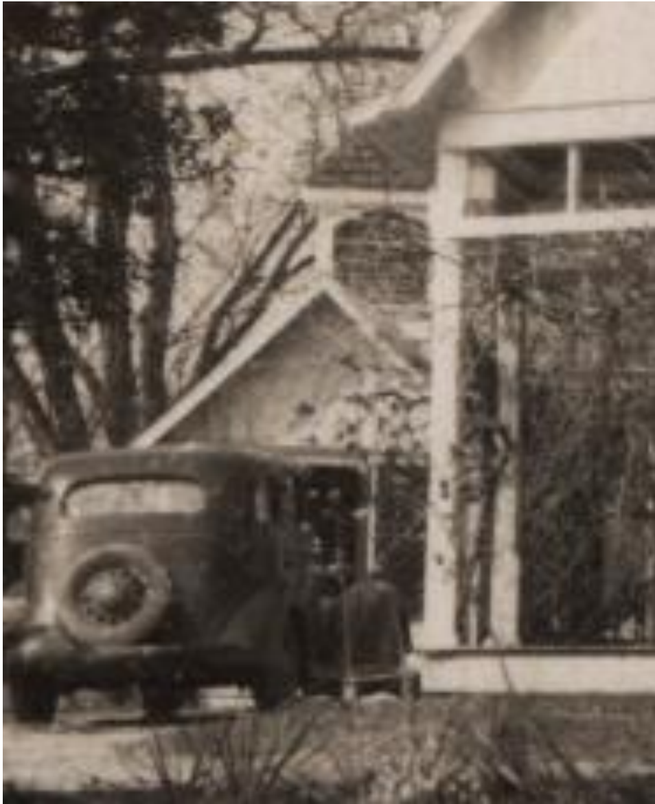
Figure 5: View of secondary building, ca. 1945.
