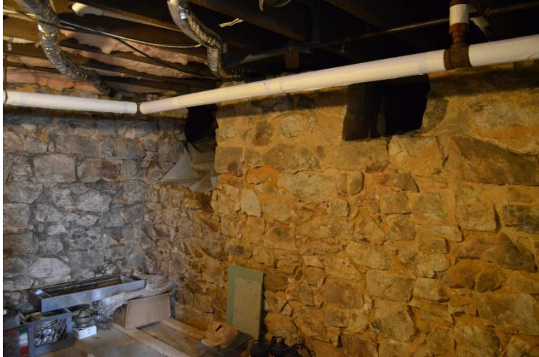
Figure 37: View of the stone foundation in the original I-house looking east towards crawl space under the front gable addition.
