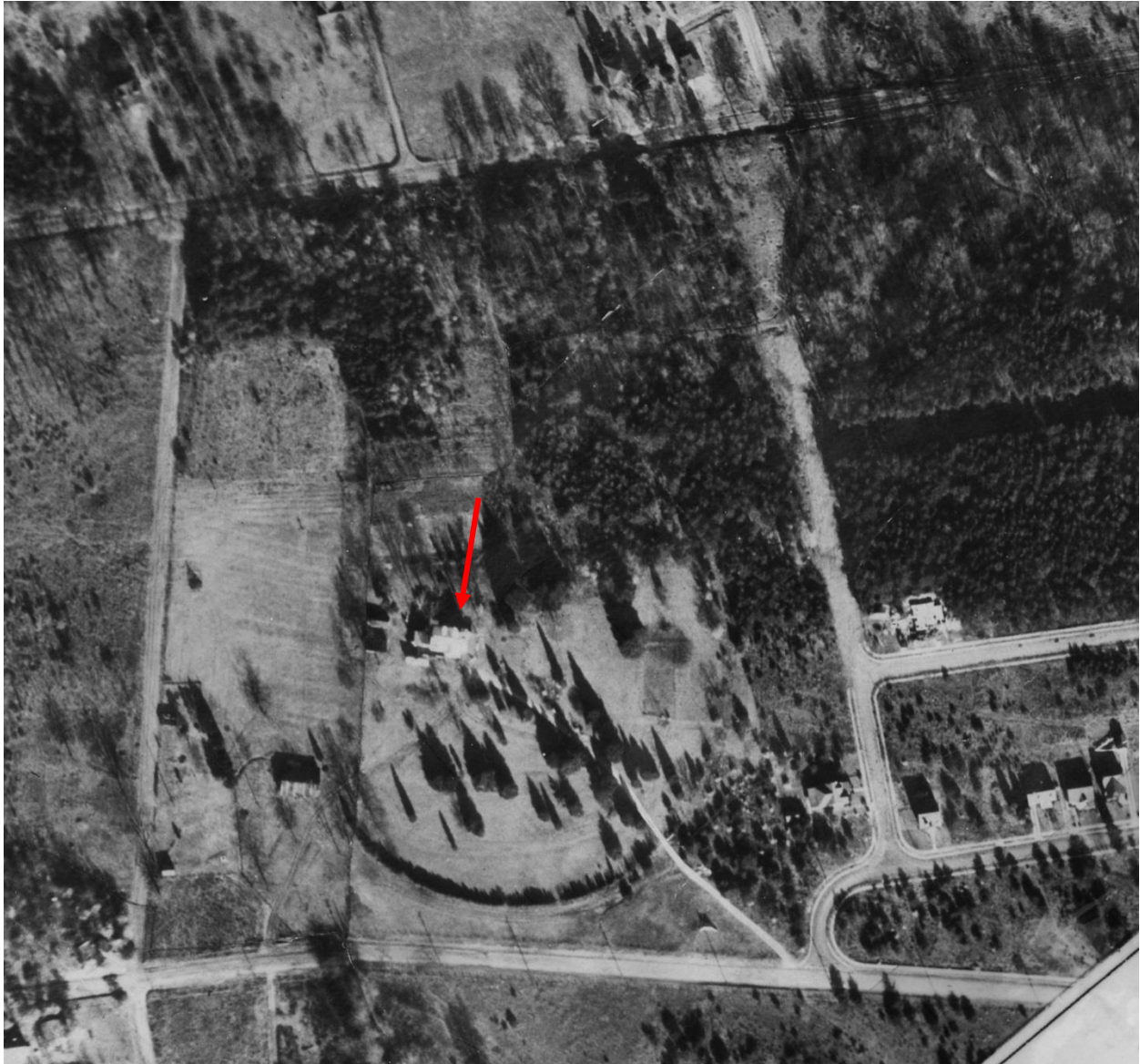
Figure 2: View of Broadview, 1934. The red arrow points to the house. Source: Aerial Photographic Map of Arlington County, Virginia . January 11, 1934, Sheet 23, Arlington County GIS.
