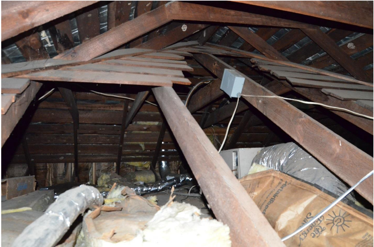
Figure 13: View of the remaining parts of the I-house's eastern slope of its side gable roof.
