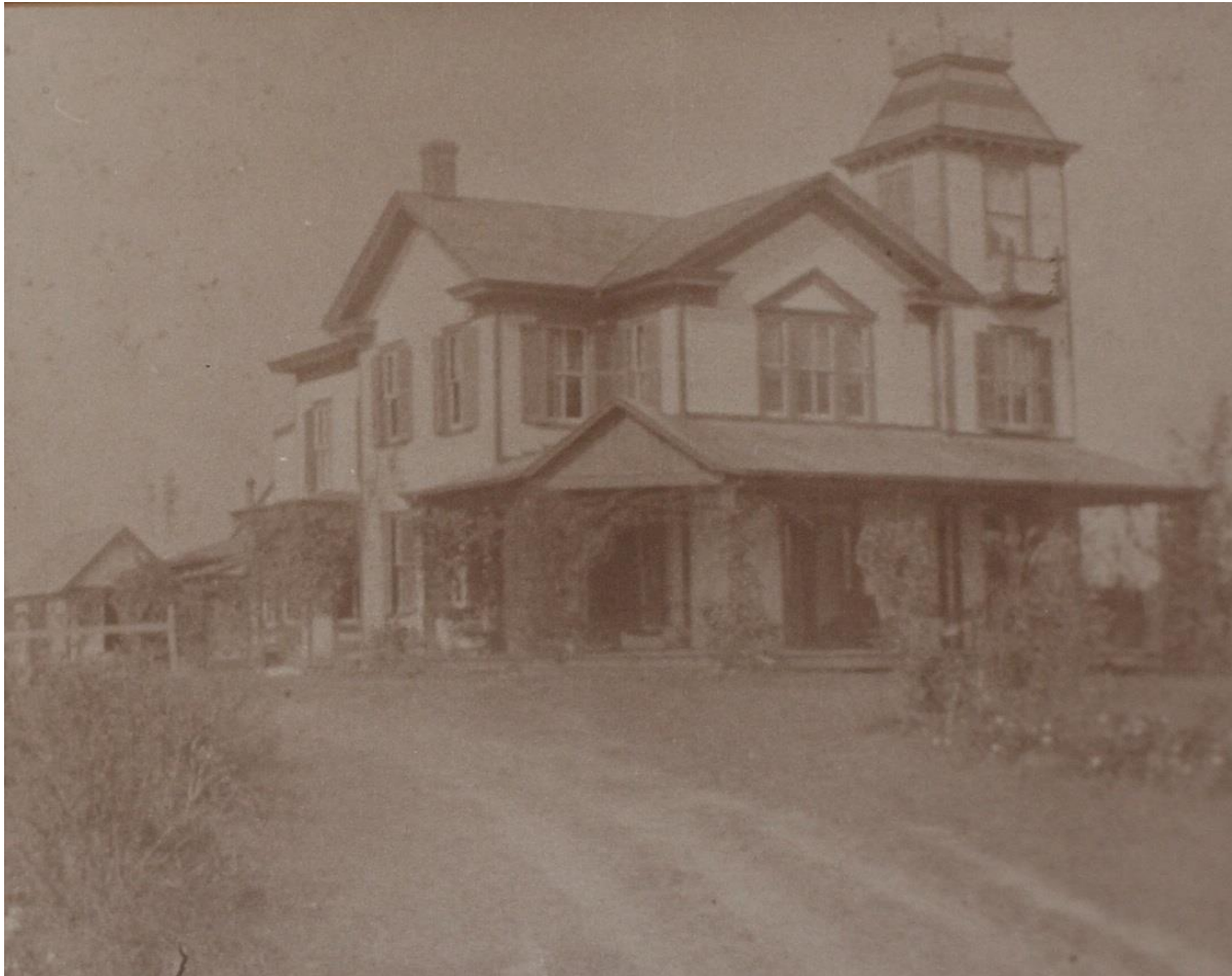
Figure 1: View of Broadview looking northwest at main façade, early-twentieth century. Source: Angela Guzman and Alex Deucher, the current owners of Broadview.
