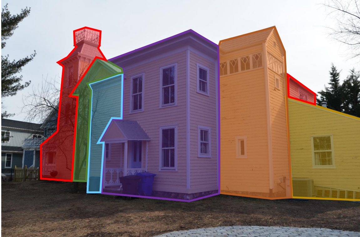
Figure 7: View of north elevation looking southeast from the subject property. On the lower image, the shaded portions are as follows: 1) the green is the original I-house (1881); 2) the red is the three-story front tower and rear shed roof addition (ca. 1898); 3) the yellow is the one-story kitchen addition (1900-1934); 4) the light blue is the two-story shed roof bathroom addition (1900-1934); 5) the purple is the two-story flat-roof addition (1900-1934), and 6) the orange is the gabled-roof tower addition (ca. 1990).
