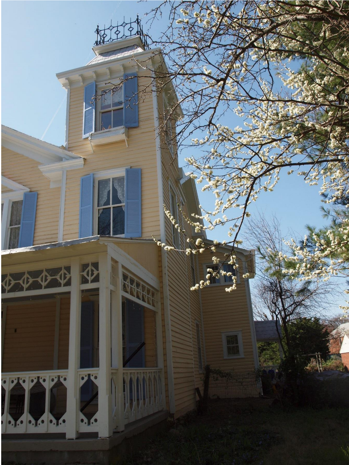
Figure 8: View of the east and north elevations looking west from the subject property. *Photograph taken by Cynthia Liccese-Torres, 2012.
