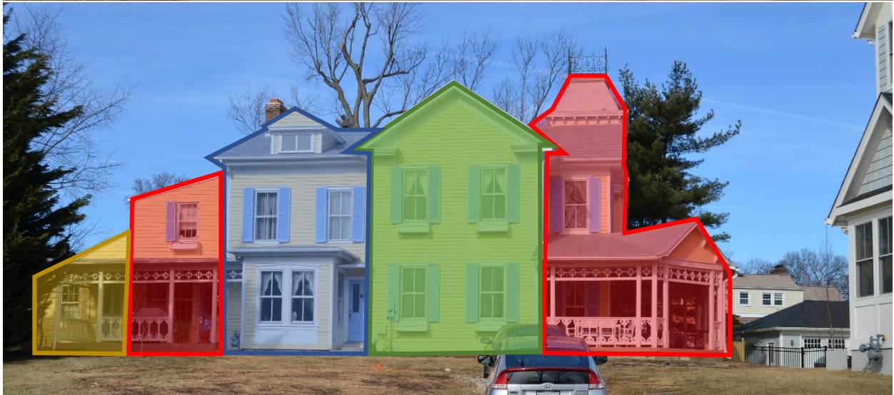
Figure 4: View of the south elevation of Broadview looking north from 14 th Street. On the lower image, the shaded portions are as follows: 1) the green is the original I-house (1881); 2) the blue is the rear gable addition (ca. 1886); 3) the red is the front gable addition and the rear two-story shed roof addition (ca. 1898); and 4) the yellow is the one-story shed addition (1900-1934).
