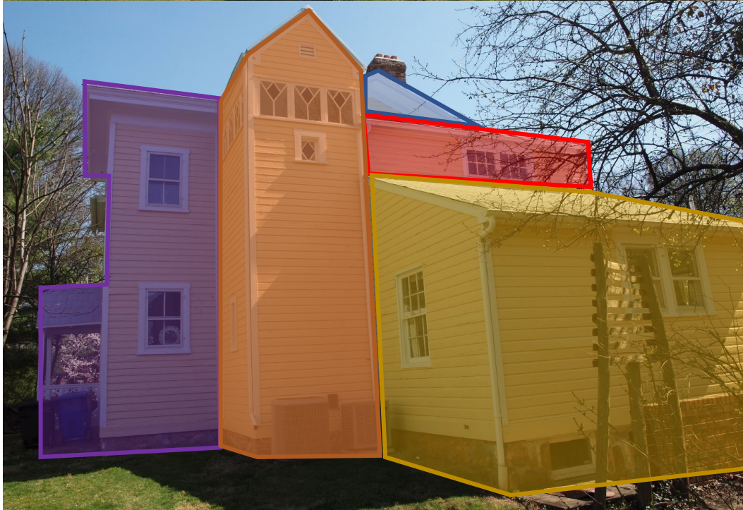
Figure 6: View of west elevation looking east from subject property. On the lower image, the shaded portions are as follows: 1) the blue is the rear gable roof addition (ca. 1885); 2) the red is the two-story shed roof addition (ca. 1898); 3) the yellow is the one-story kitchen addition (1900-1934); 4) the purple is the flat roof addition (1900-1934); 5) and the orange is the gabled-roof tower addition (ca. 1990).
