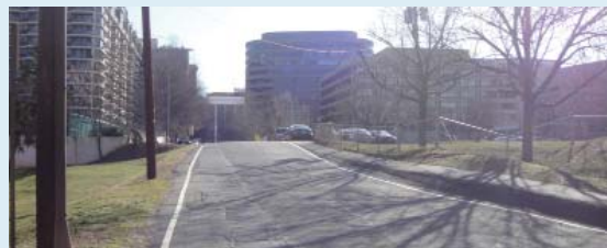
18th Street, seen looking east from North Quinn Street, has no sidewalk on its north side (left) and a makeshift asphalt sidewalk on its south side (right).
