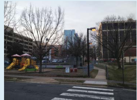
A path connects 18th Street (in foreground) to Wilson Boulevard past Rosslyn Highlands Park and Fire Station 10. Note misalignment of the curb cut with crosswalk and path.
