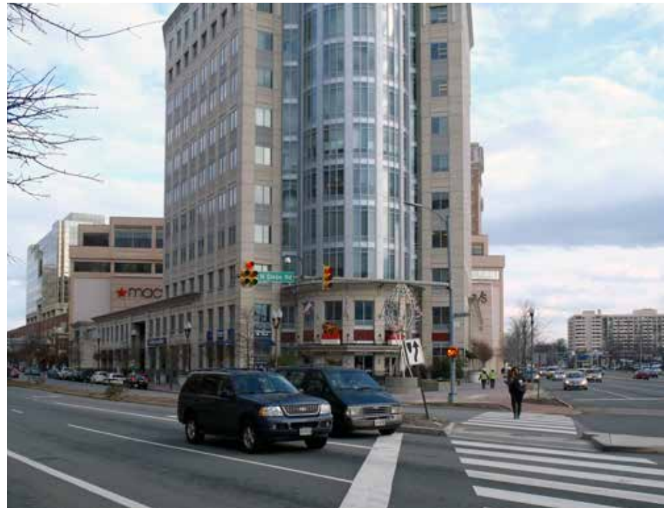
3. Existing Wilson Blvd. Facade - West Elevation
