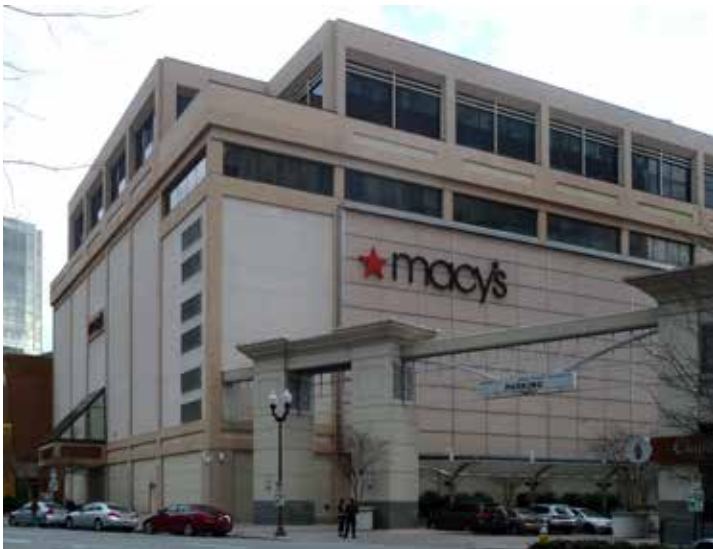
Existing View - NW Corner
