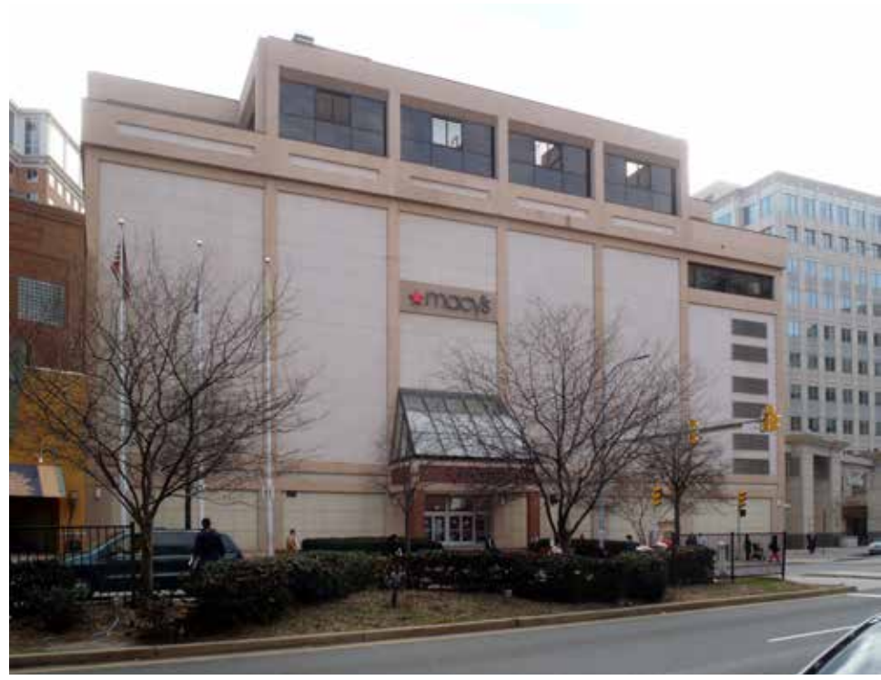
1. Existing Wilson Blvd. Facade - North Elevation
