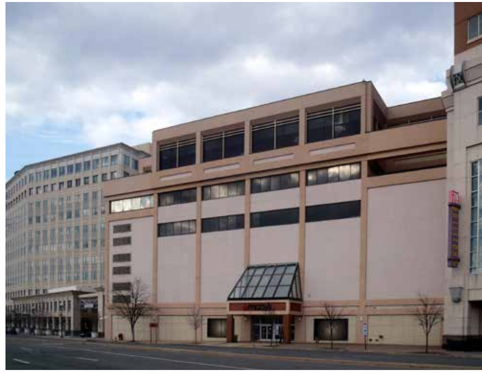
2. Existing Glebe Road Facade - South Elevation
