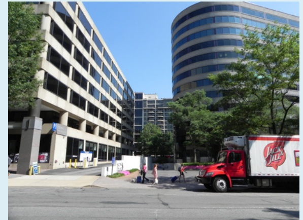
View of 1555 Wilson Boulevard looking North and West
