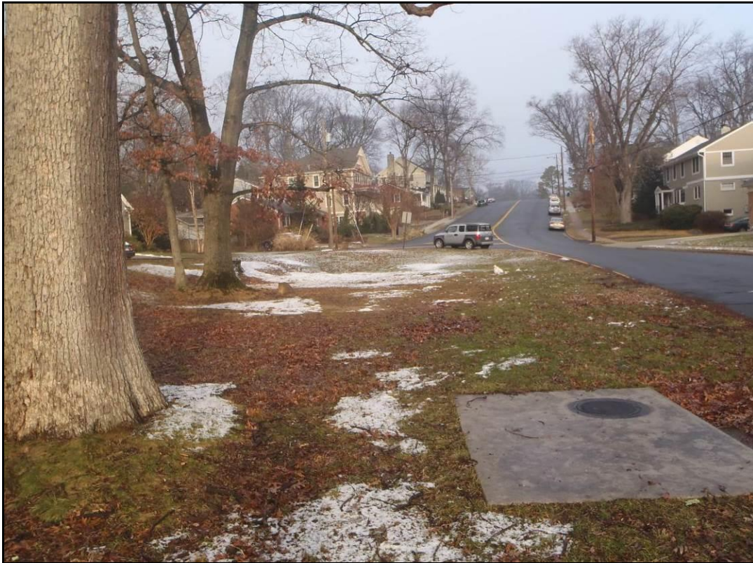
Photo 2: Overview of Project Area Showing Storm Water Drain, Facing North.
