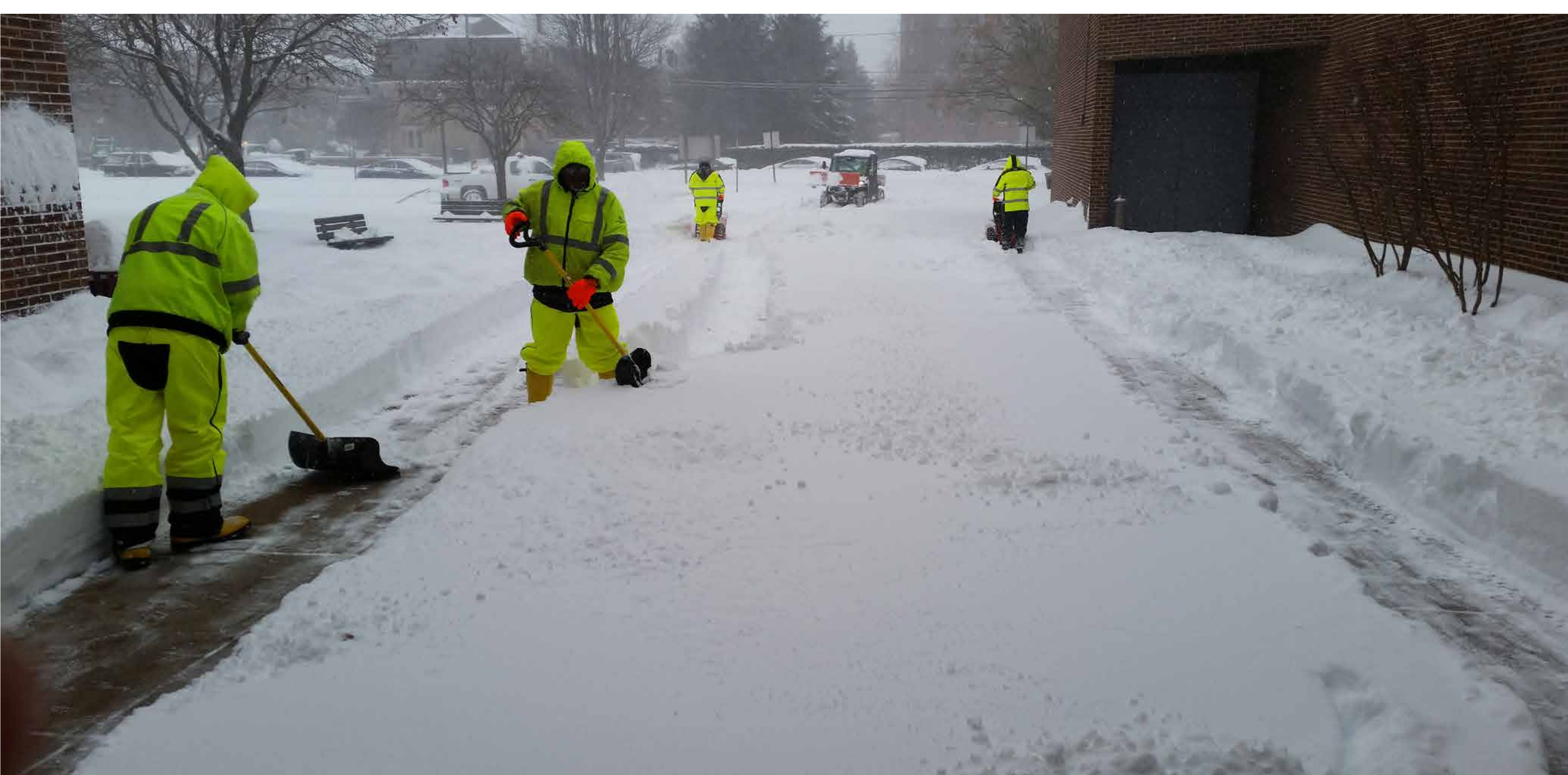
Clearing snow at T.J.
