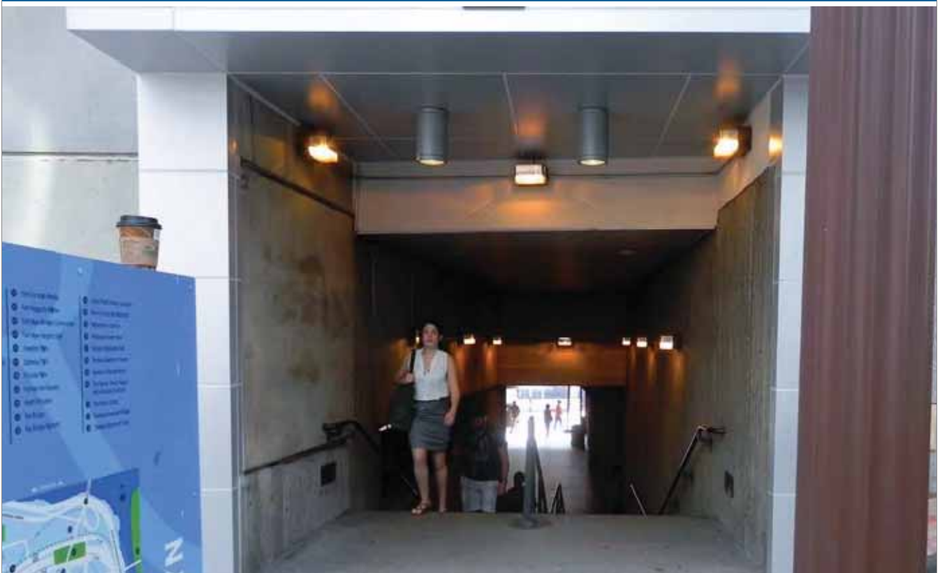
Metro Station Entrance from Fort Myer Drive
