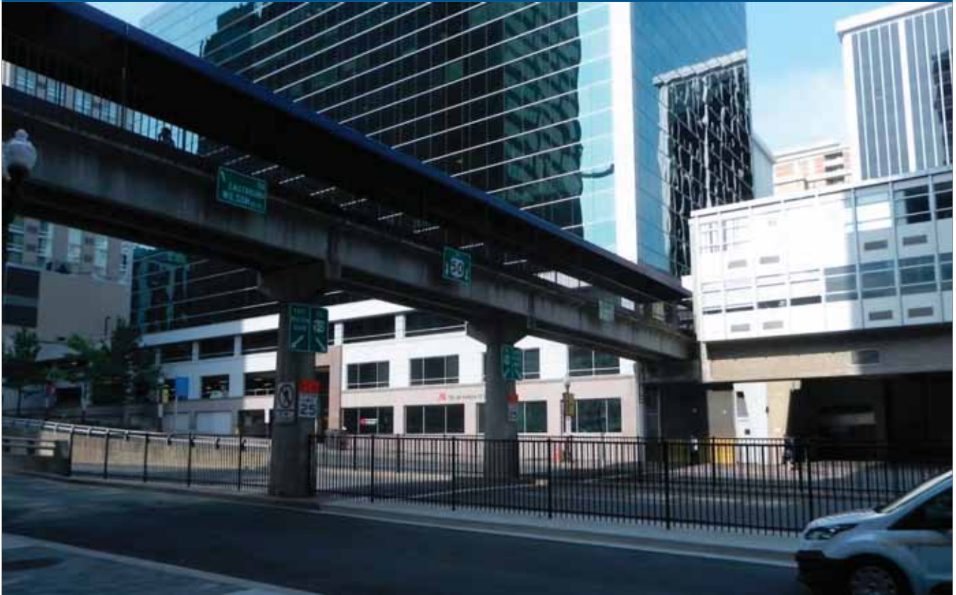
Fort Myer Drive, mid-block between Wilson and 19 th Street
