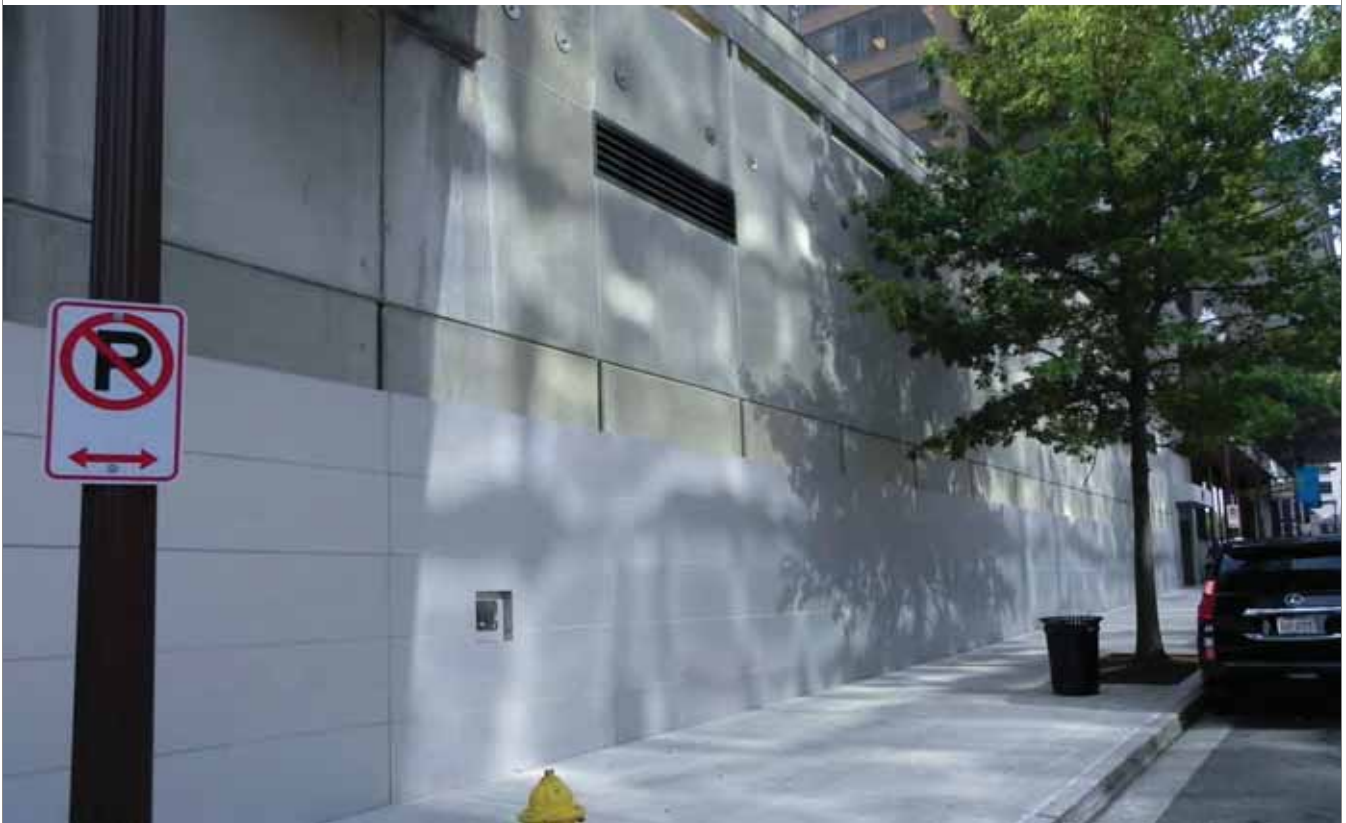
Metro Station Façade along Fort Myer Drive
