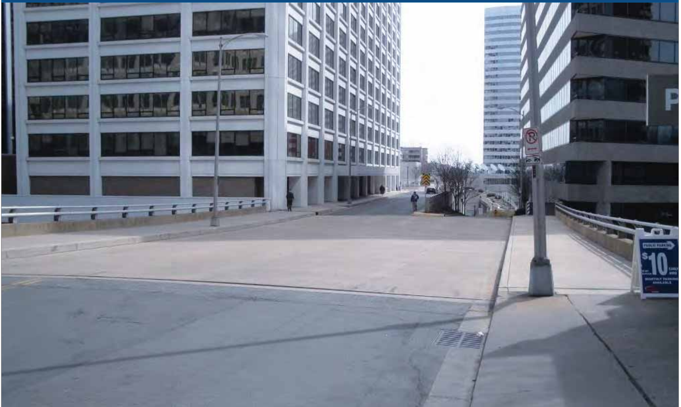
View of 17 th Street looking east near bridge over Fort Myer Drive
