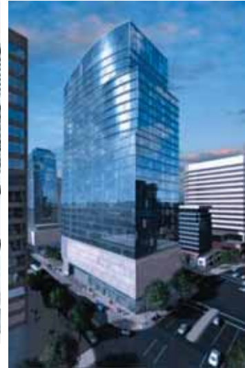
Approved Central Place site plan, under construction
