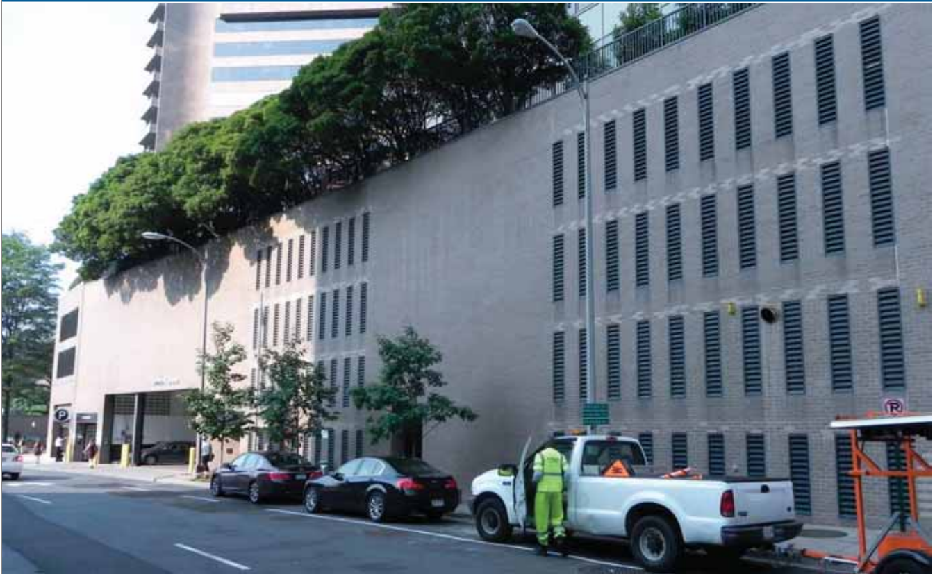
Fort Myer Drive Streetscape/Ground Plane
