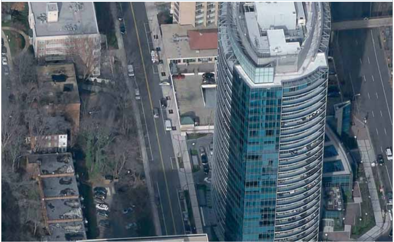
Turnberry Tower and abrupt Nash Street transition
