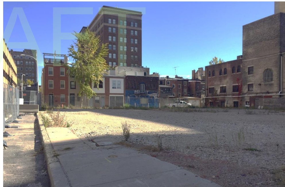
Same lot prepped for construction, fall 2016
