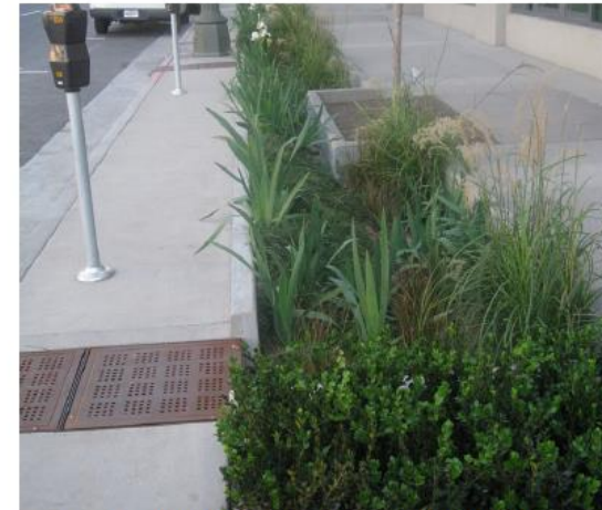
Green infrastructure like this stormwater planter serves double-duty as streetscape beautification and natural stormwater management.
