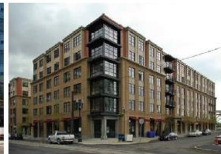
Intermediate cornice + material change
