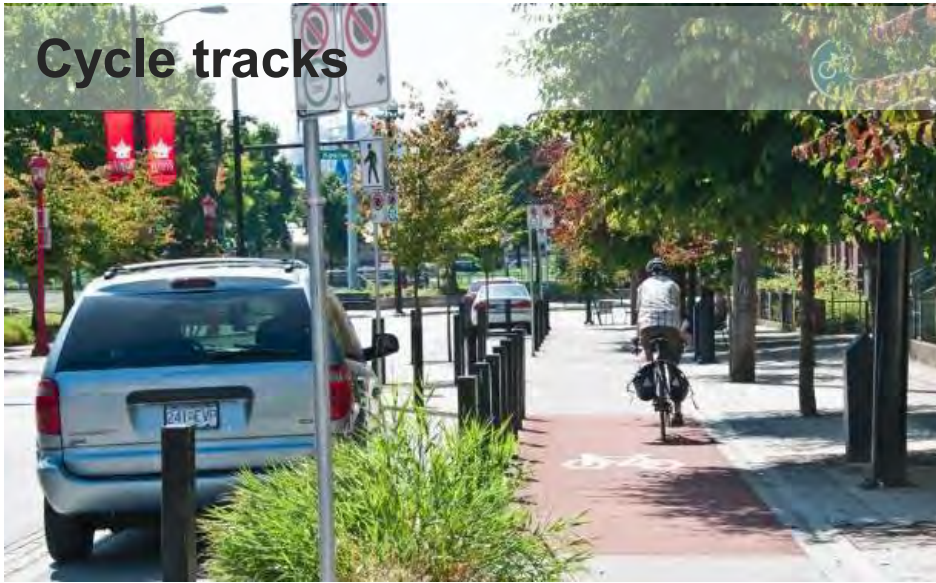
Pathway bridges over roadways
