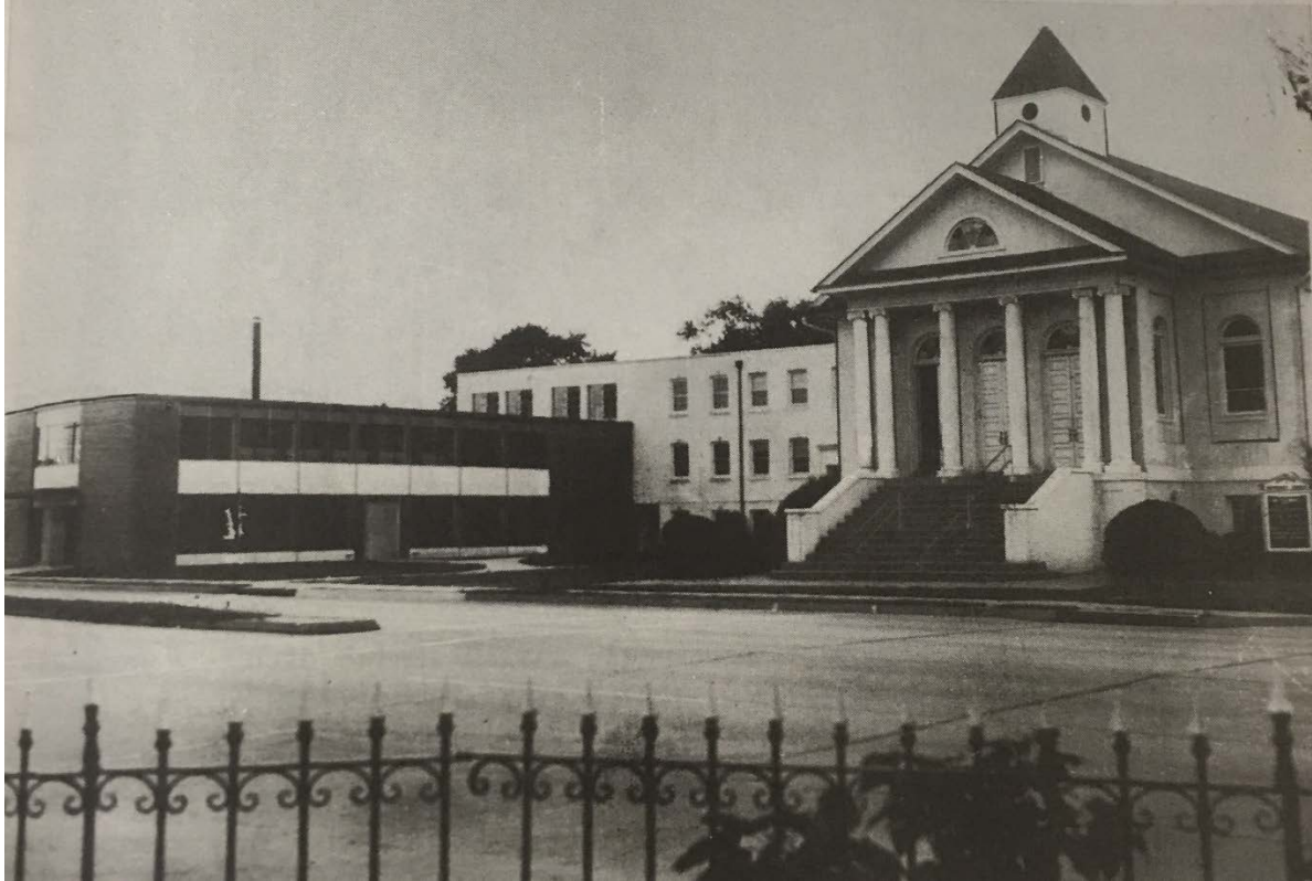
Figure 8: View of the Central United Methodist Church, ca 1955, showing the new youth center off the education wing.
