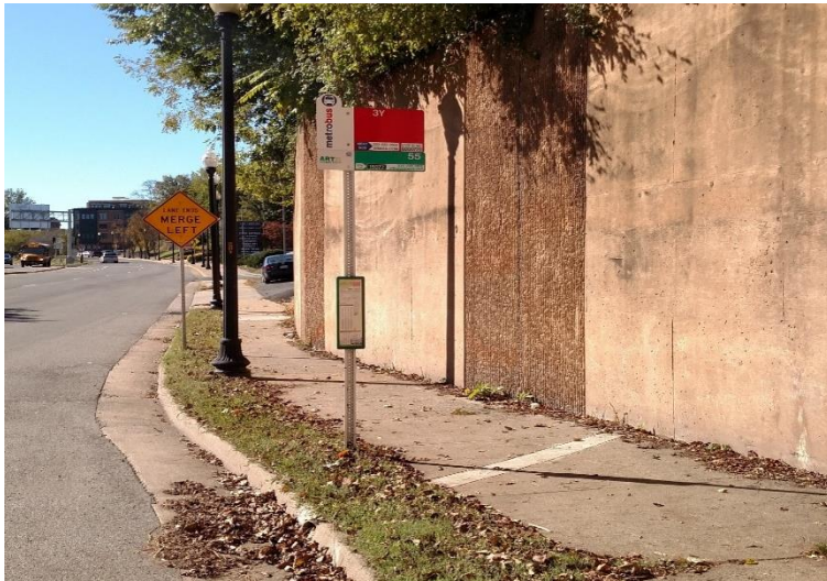
I-66 – Lacks Accessibility. Not ADA Compliant
