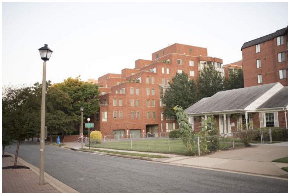
VIEW DOWN 11TH STREET SOUTH EAST
