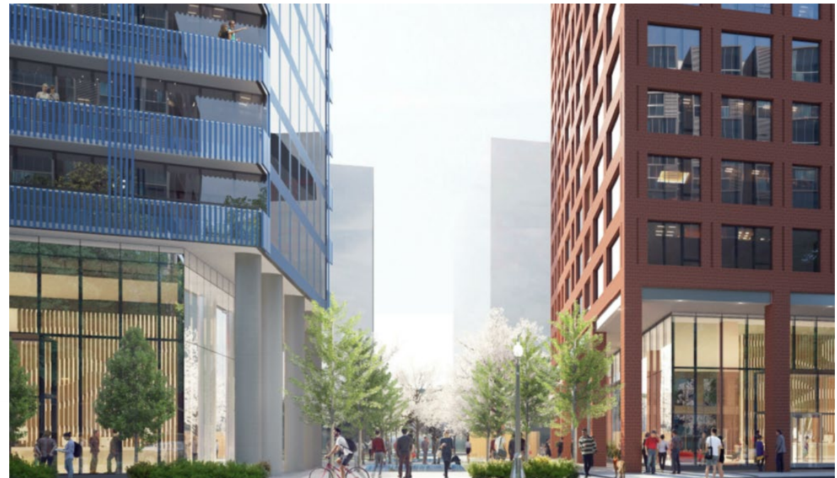
East-west ped. path (looking west)
