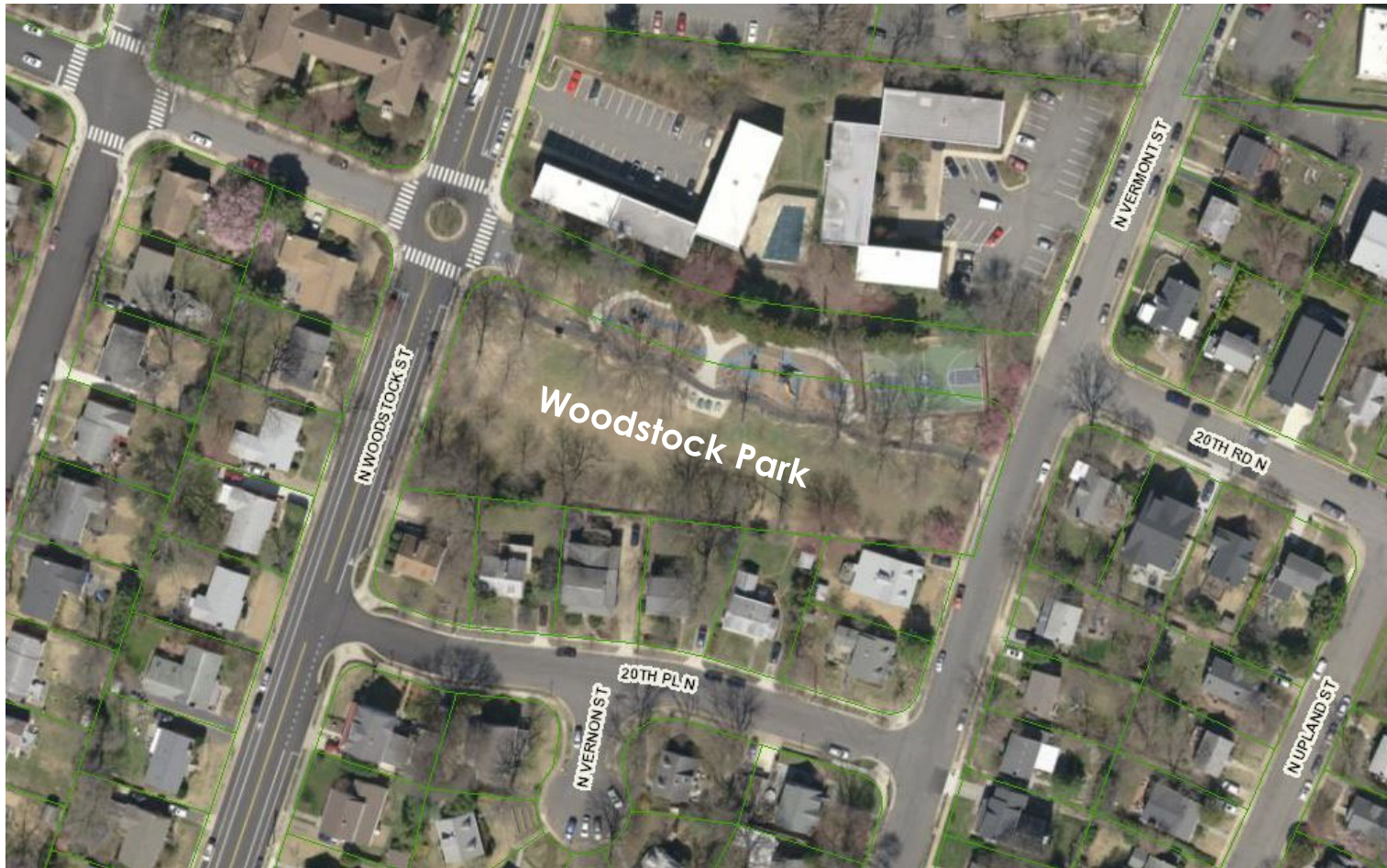
Woodstock Park Stormwater Detention Vault
