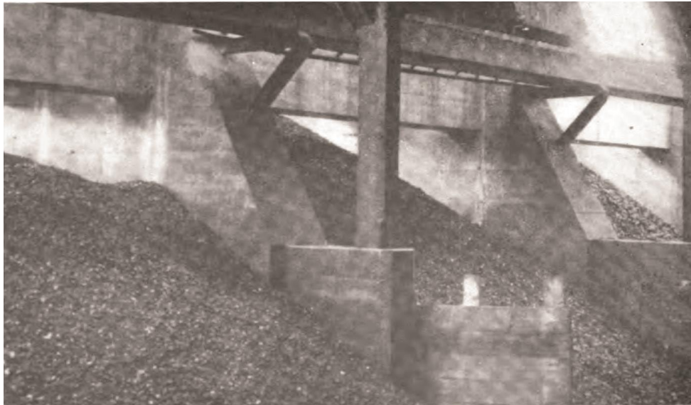
Figure 6: Doylestown, PA. View of Concrete Coal Bins and Brackets Supporting Trestle, 1910. This example is similar in design to Elliott's coal trestle.
