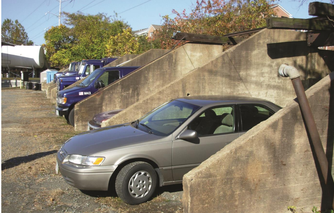
Figure 26: Looking northwest towards coal trestle from subject property. Source: Darren Hannabass.
