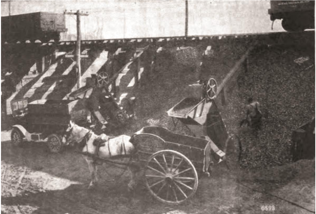
Figure 7: A Link Belt Portable Wagon Loader in Operation, circa 1915. The wooden coal pocket and bins are similar in design to Elliott's concrete trestle. Note the worker shoveling coal into the wagon loader. Source: The Grain and Feed Review, "Modern Methods of Handling Coal," The Grain and Feed Review 4 (1915): 94.
