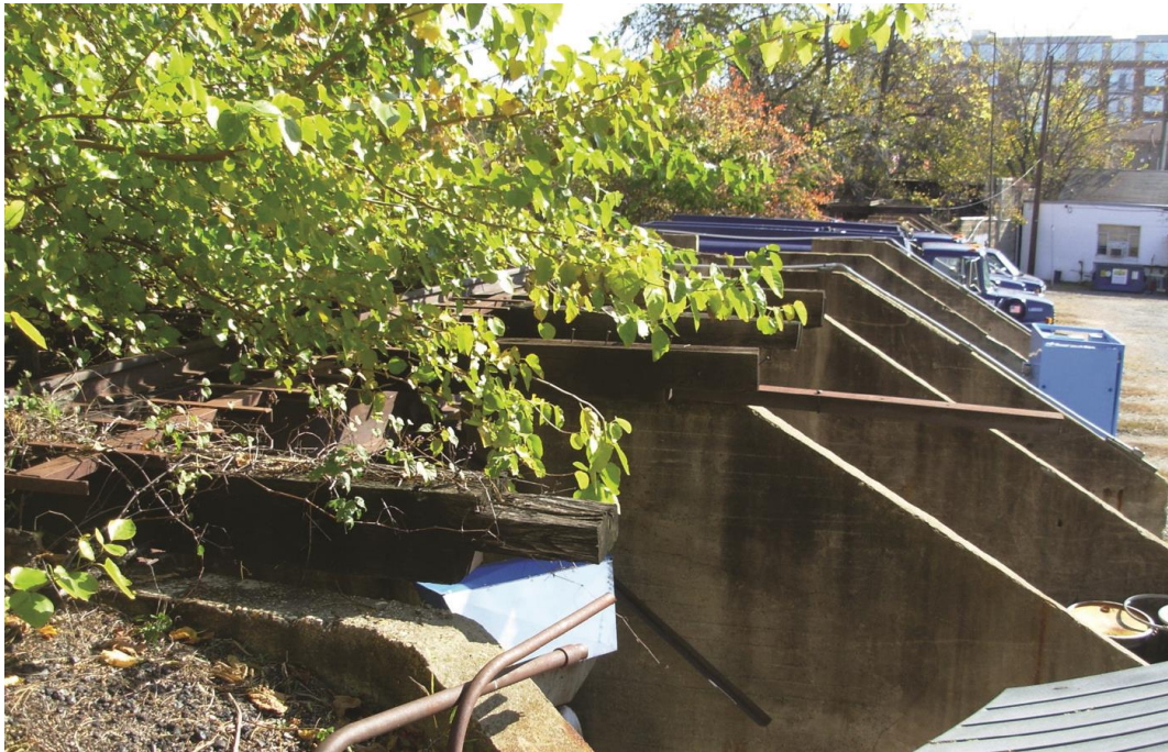
Figure 29: Looking southeast towards coal trestle from subject property. Source: Darren Hannabass.
