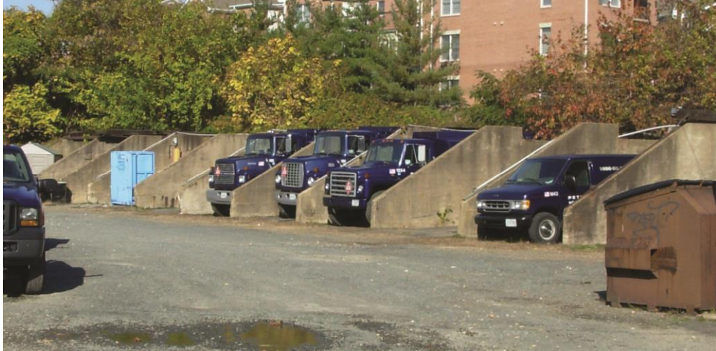
Figure 15: Benjamin Elliott's Coal Trestle, 2010. Shreve Oil Company trucks now park in between the concrete piers. The tracks were removed for this purpose. Source: Darren Hannabass.
