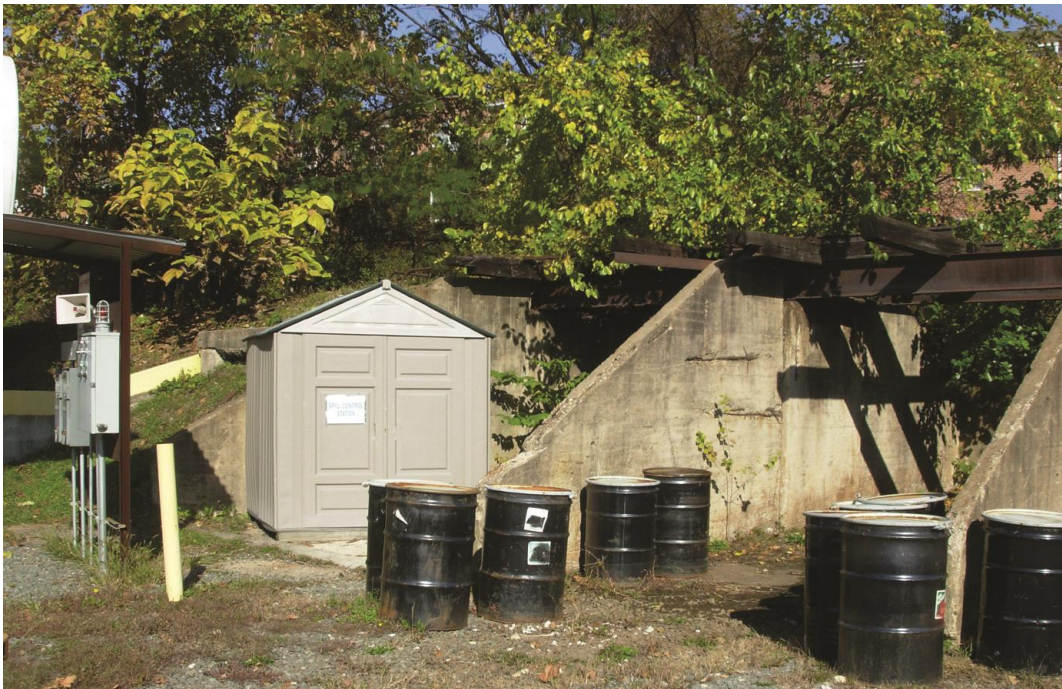
Figure 27: Looking northwest towards coal trestle from subject property. Source: Darren Hannabass.
