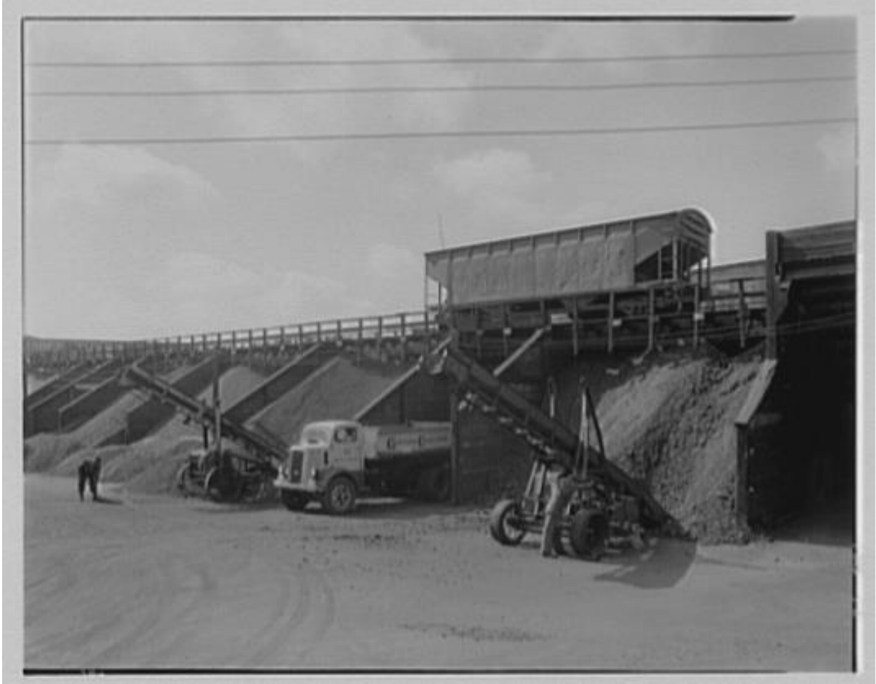
Figure 8: Griffith Coal Bin, Rosslyn, Virginia, 1947. Note the mechanical coal conveyors and the hopper car. The trestle and bins, constructed of wood, are similar in design and function to Elliott's coal trestle.
