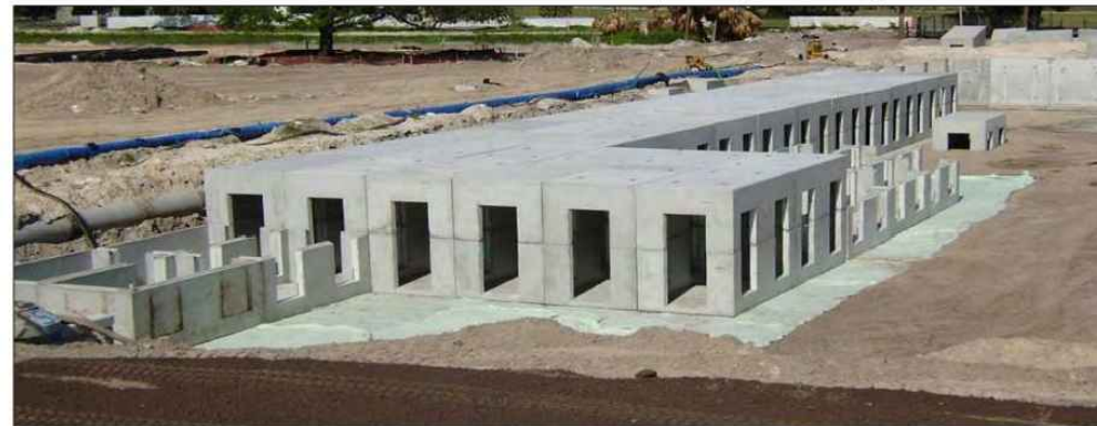
StormCapture System During Installation Process
