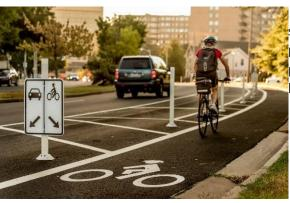
Protected bike lanes, also known as cycletracks or separated bike lanes, provide physical separation between people on bikes and motor vehicles. The separation can be provided in a number of ways including: plastic bollards, landscaping or large planters, curbs or even car parking.
